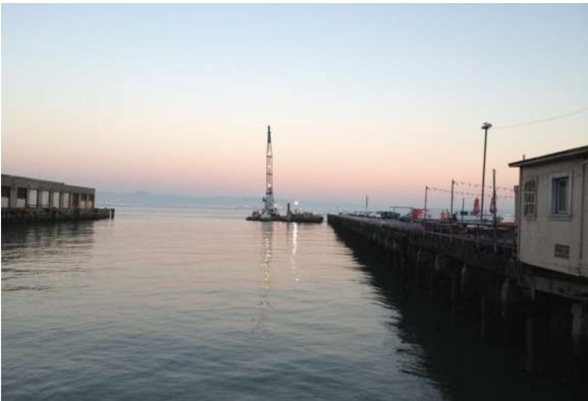
Figure 2 – Vortex set-up at HDD North Pier 30/32. View east, January 22, 2015.
