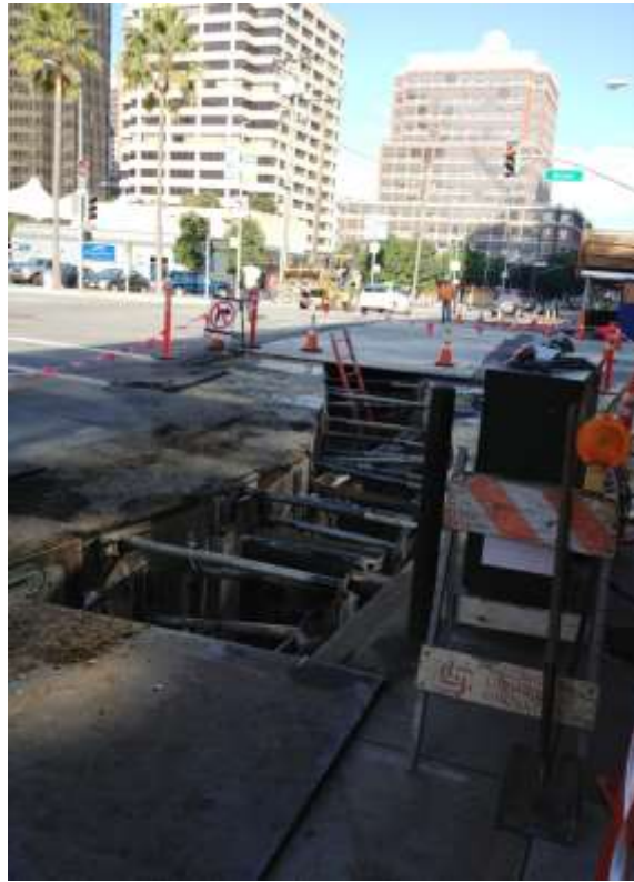
Figure 3 – Underground duct bank potholing on Folsom Street. View north, January 22, 2015.
