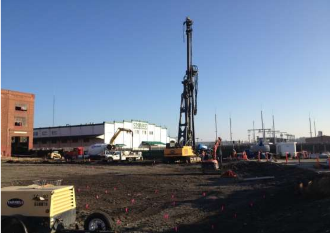
Figure 1 – Drill displacement columns being installed at Potrero Switchyard. View south, January 22, 2015.
