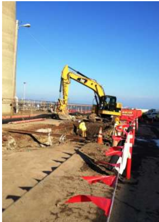
Figure 4 – Underground duct bank excavation on 23 rd Street. View east, January 22, 2015.
