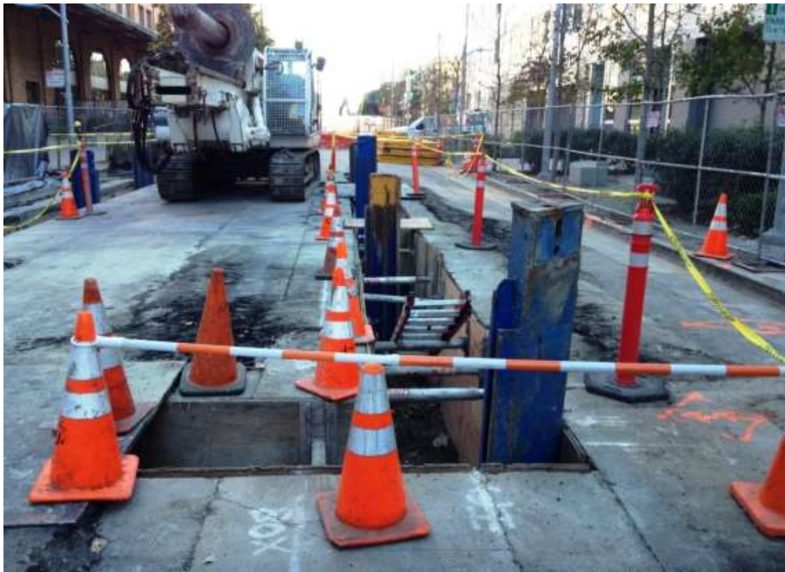
Figure 3 – Vault shoring work on Spear Street. View southeast, February 20, 2015.
