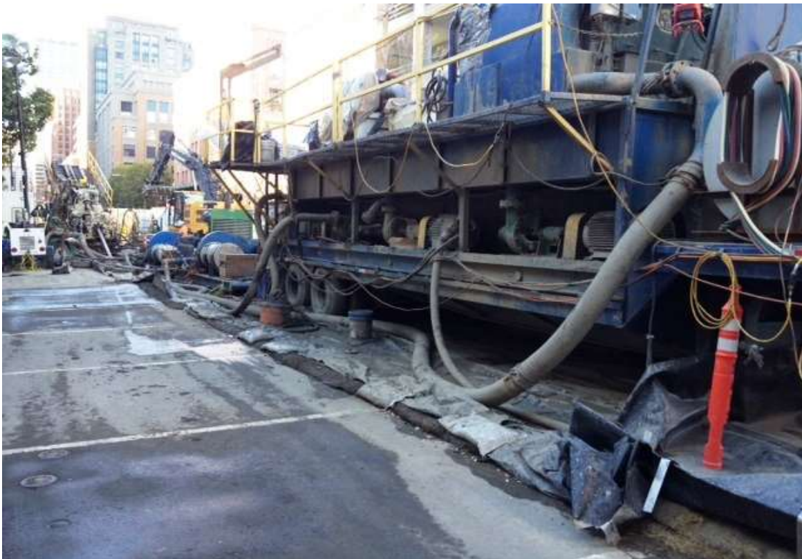
Figure 2 – HDD Company drilling at HDD North. View northwest, February 20, 2015.
