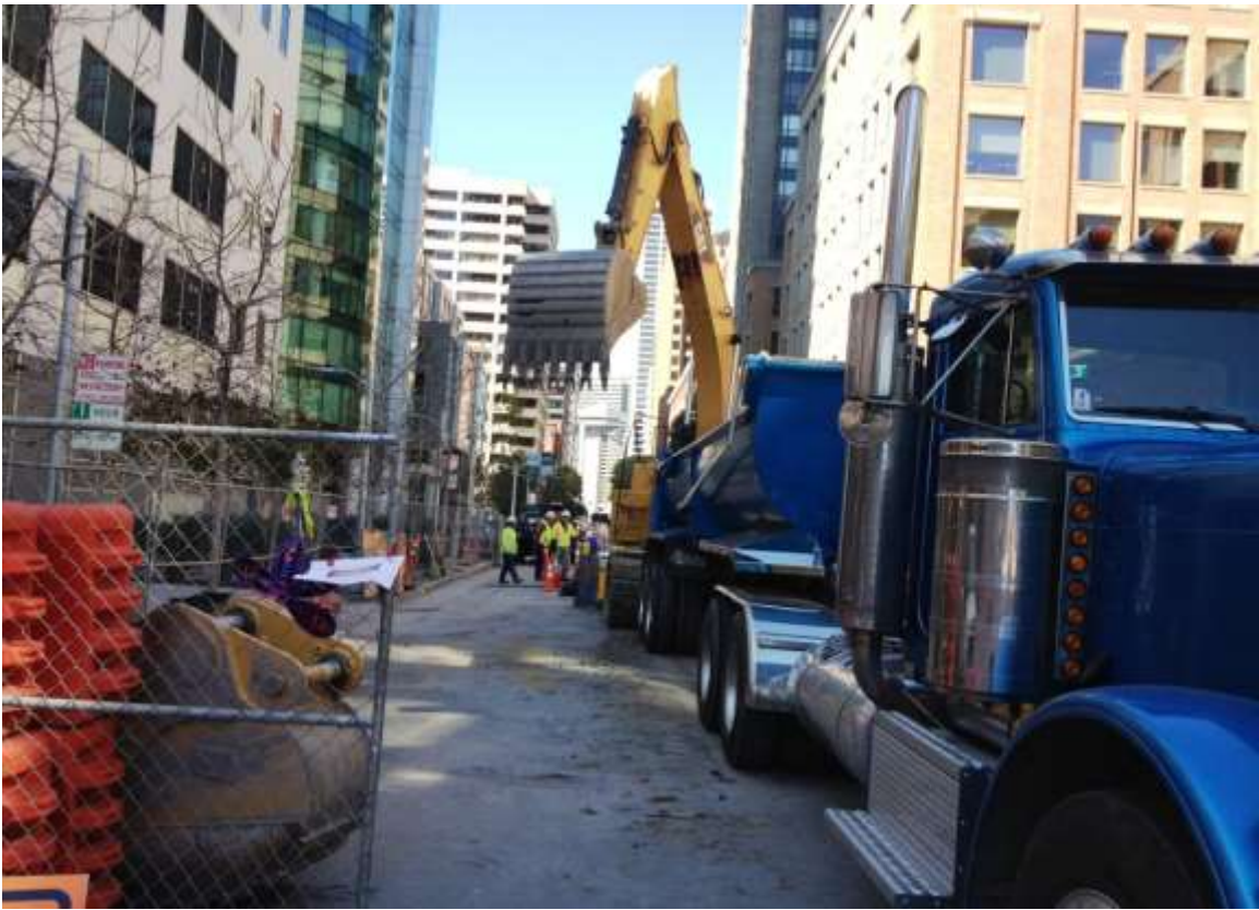
Figure 3 – Excavating for vault on Spear Street. View west, March 4, 2015.
