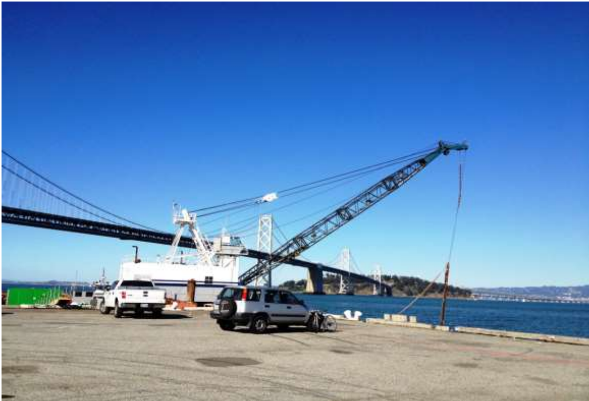
Figure 2 – Vortex set-up at HDD North – Pier 30/32. View north, March 4, 2015.
