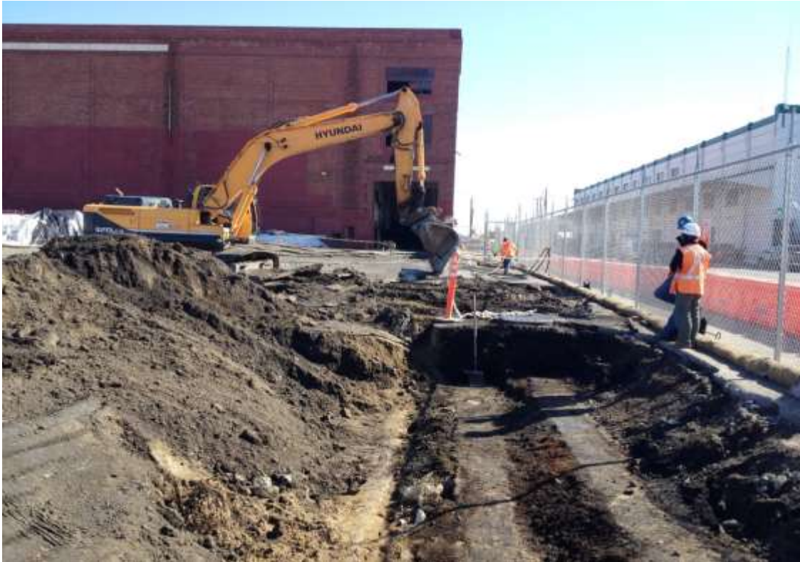
Figure 1 – Demolition of sidewalk at Potrero Switchyard, view east, March 4, 2015.
