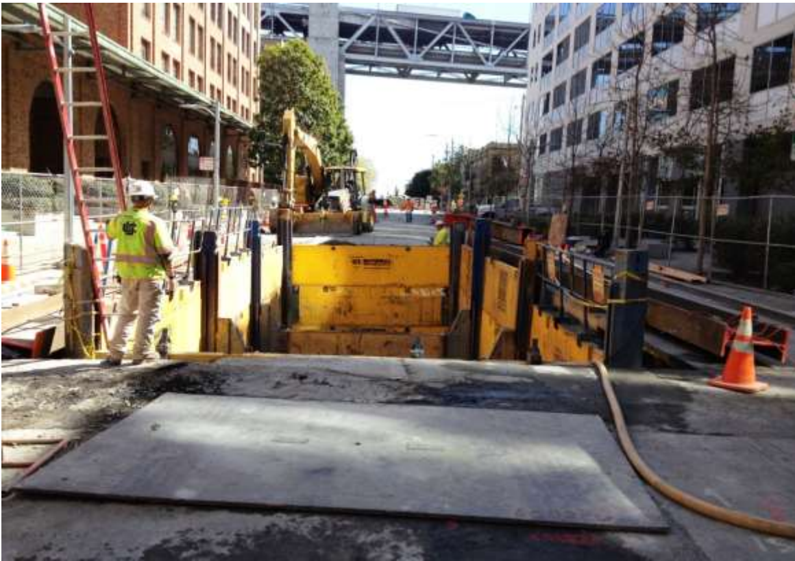
Figure 3 – Vault excavation on Spear Street. View east, March 12, 2015.
