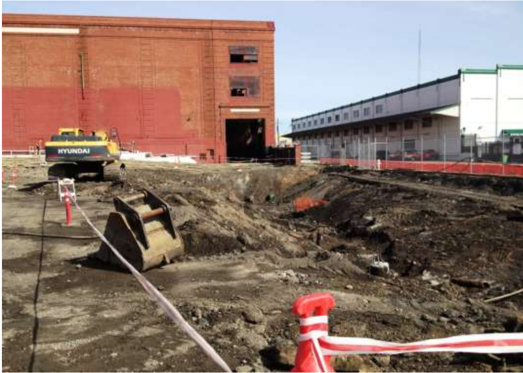
Figure 1 – Excavation at Potrero Switchyard, view east, March 12, 2015.
