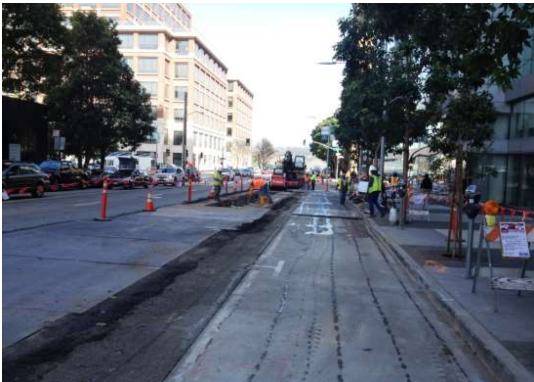
Figure 2 – Excavating duct bank on Folsom Street. View north, March 12, 2015.
