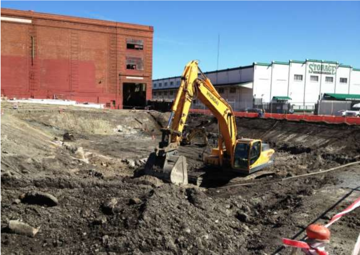
Figure 1 – Excavating at Potrero Switchyard, view southeast, March 25, 2015.
