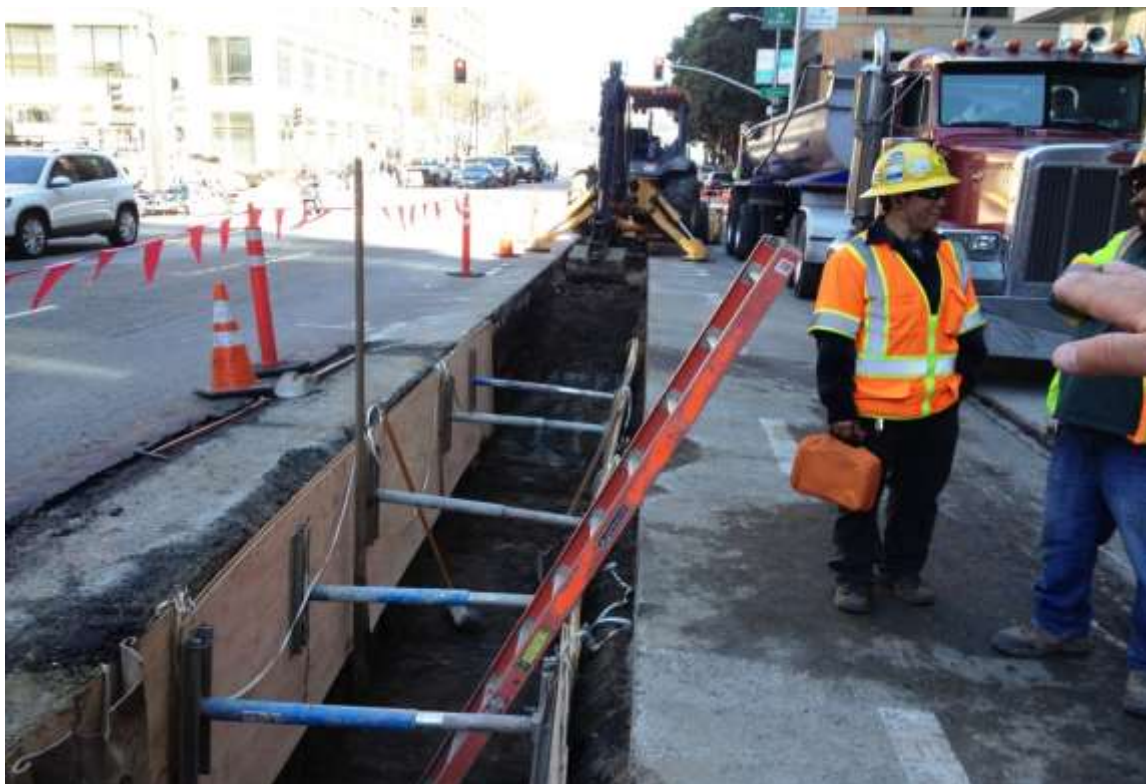
Figure 2 – Underground duct bank work on Folsom Street. View north, March 25, 2015.
