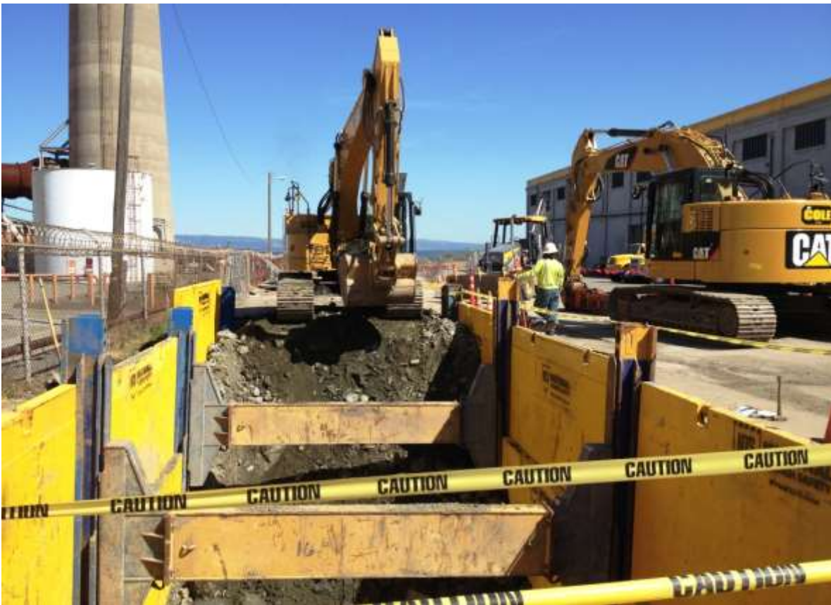
Figure 4 – Vault pit excavation on 23rd Street. View east, March 25, 2015.
