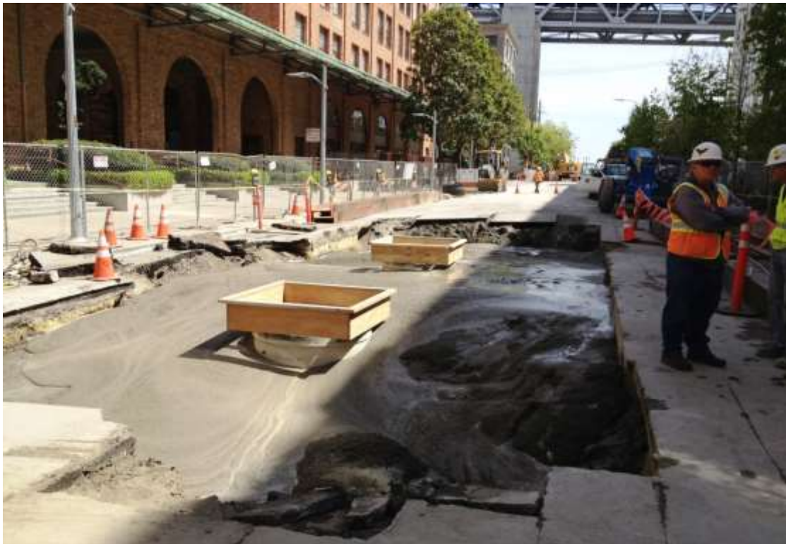
Figure 2 – Cement slurry poured over vault on Spear Street. View east, April 9, 2015.
