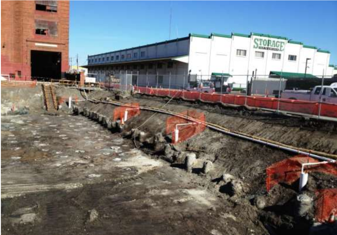
Figure 1 – Exposing pile columns at Potrero Switchyard. View southeast, April 14, 2015.
