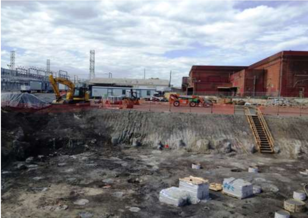
Figure 1 – Drill displacement columns (DDCs) exposed at Potrero Switchyard. View north, May 7, 2015.
