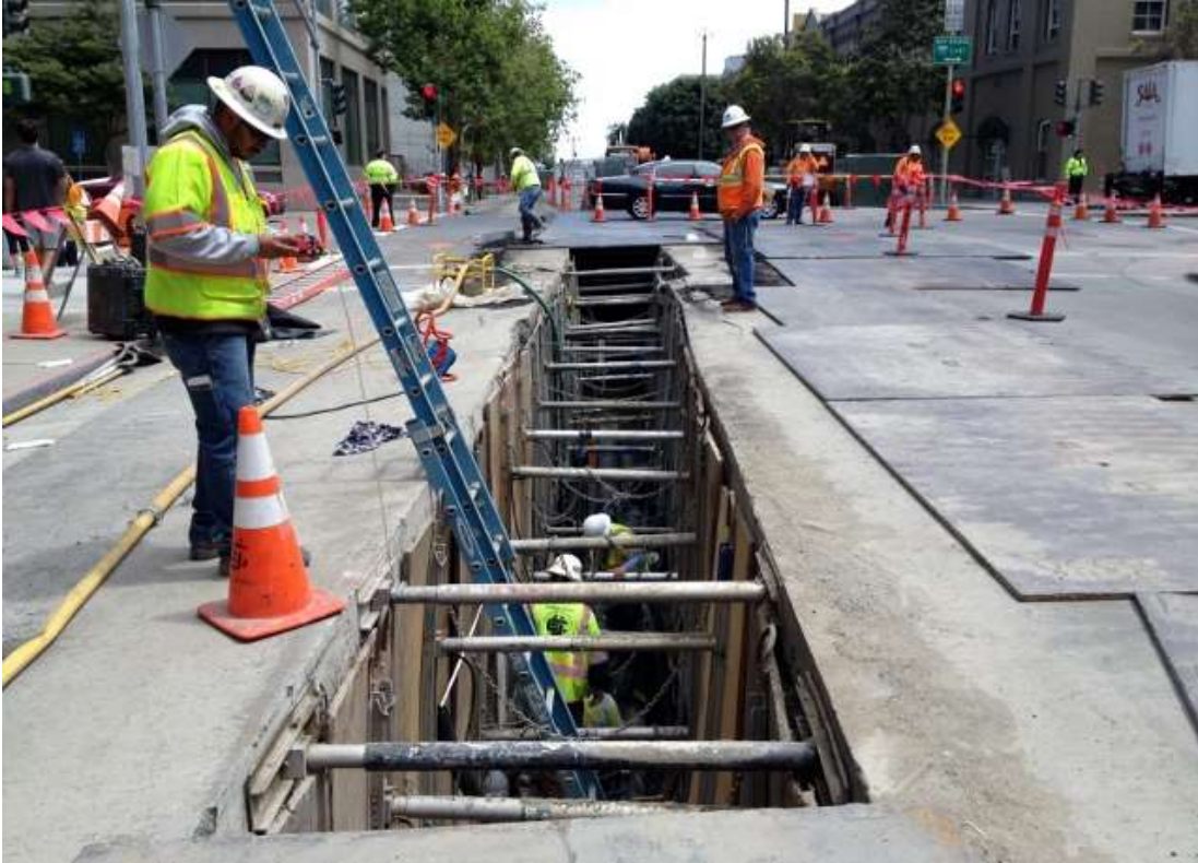
Figure 1 – Work at duct bank north on Spear Street. View east, May 15, 2015.
