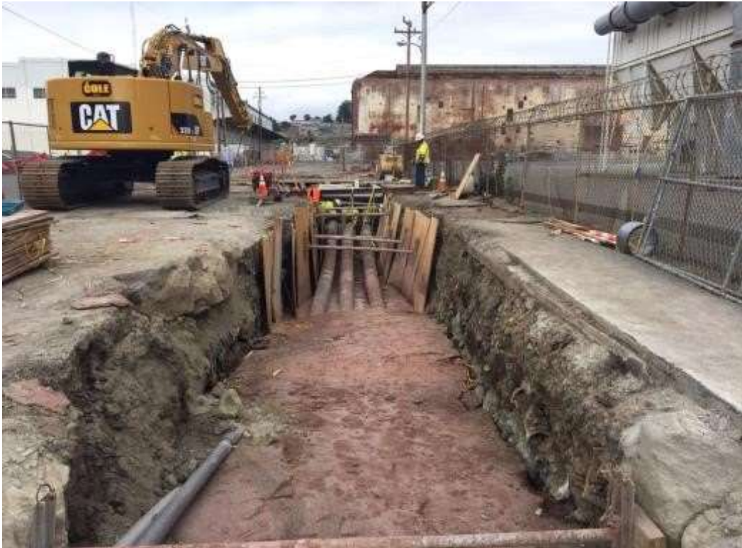
Figure 3 – Fusing duct bank conduit on 23 rd Street. View west, May 22, 2015. Photo courtesy of PG&E.
