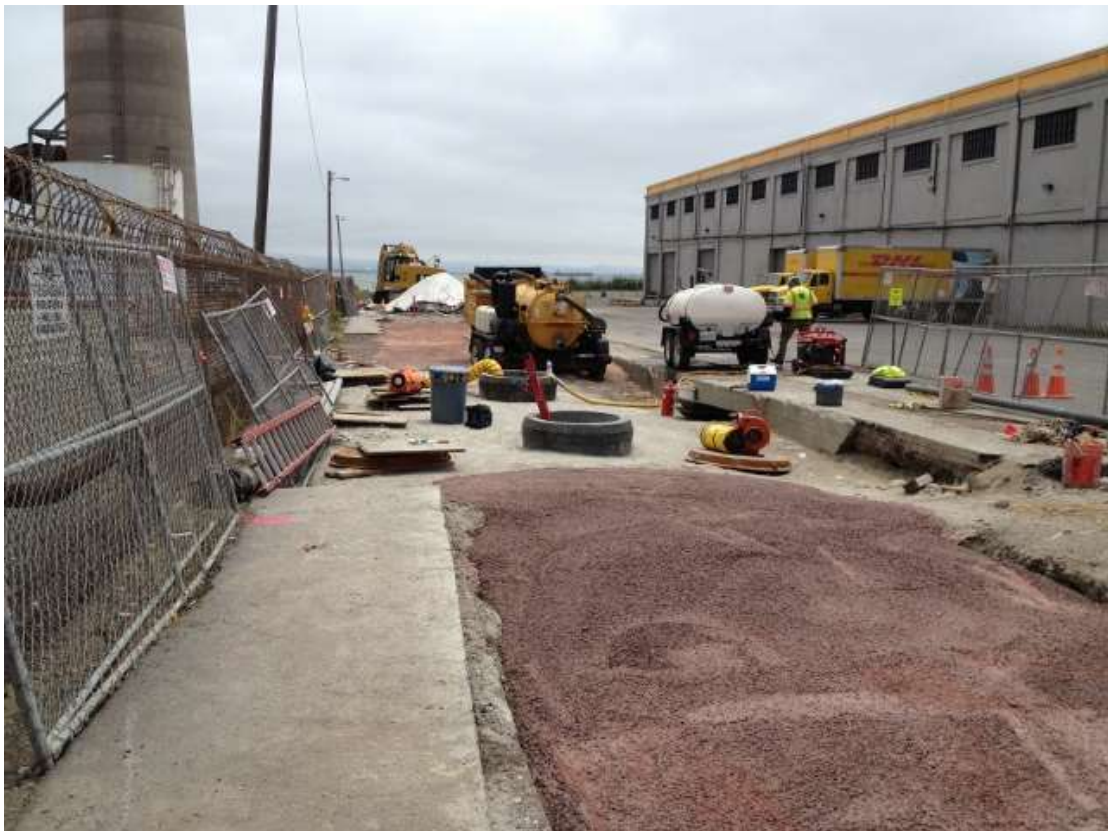
Figure 4 – Cleaning vault on 23 rd St. View east, May 28, 2015.
