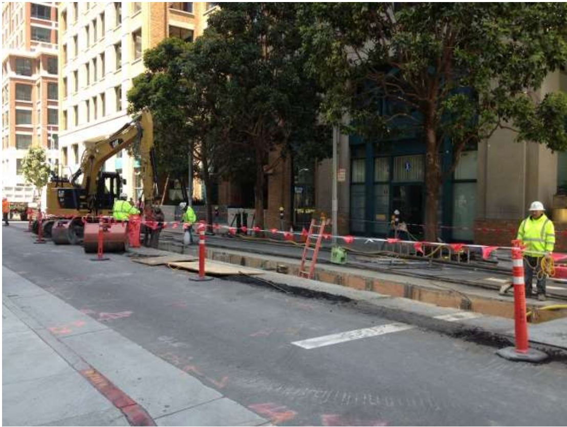
Figure 3 – Excavating duct bank trench on Spear Street. View northwest, May 28, 2015.
