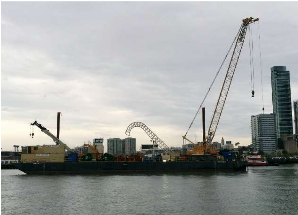
Figure 6 – Cable-laying barge anchored off Pier 30/32 in SF Bay. View southwest, June 10, 2015.
