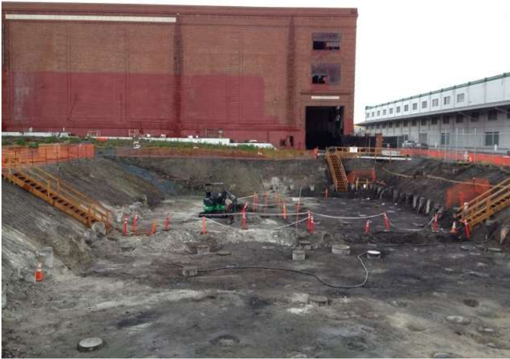
Figure 1 – Potrero Switchyard. View east, June 10, 2015.
