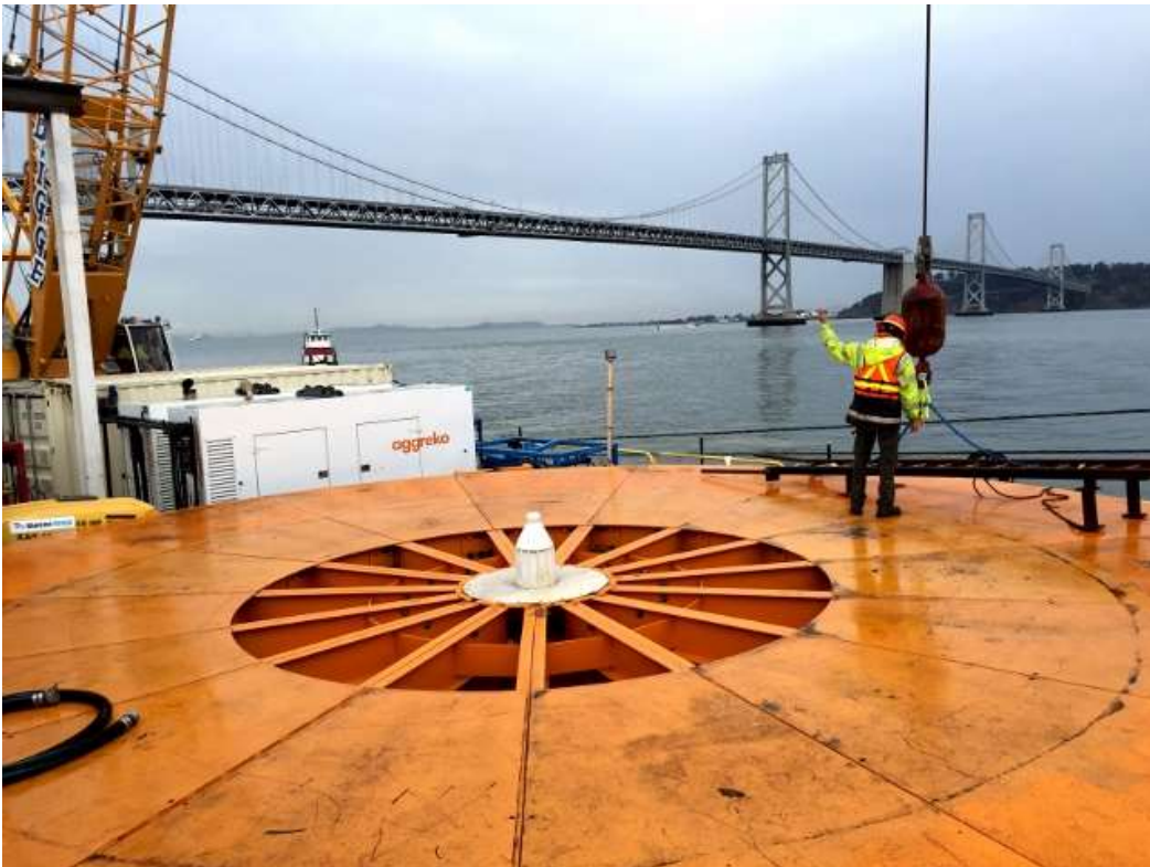
Figure 5 – Cable-laying barge tour off Pier 30/32 in SF Bay. View north, June 10, 2015.
