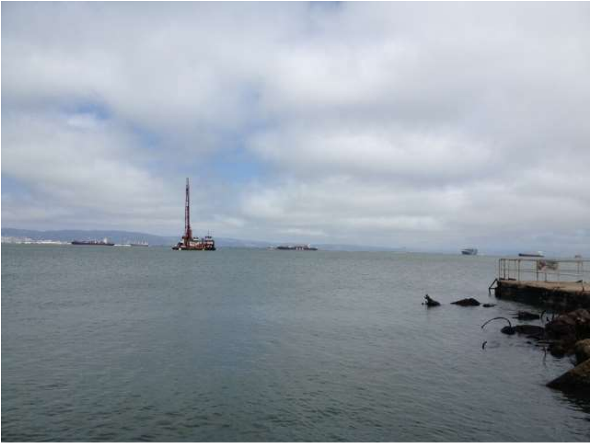
Figure 5 – Durocher at south end of project. View east, July 21, 2015
