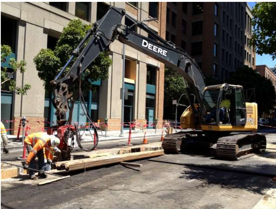
Figure 2 – Installing shoring in trench on Spear Street. View northeast, July 29, 2015.
