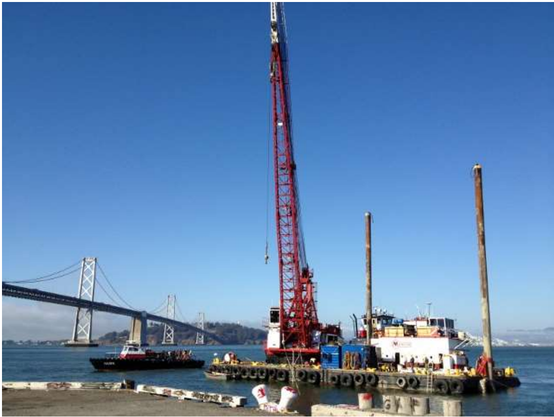
Figure 5 – Durocher at Pier 30/32 conducting diving work. View northeast, July 29, 2015
