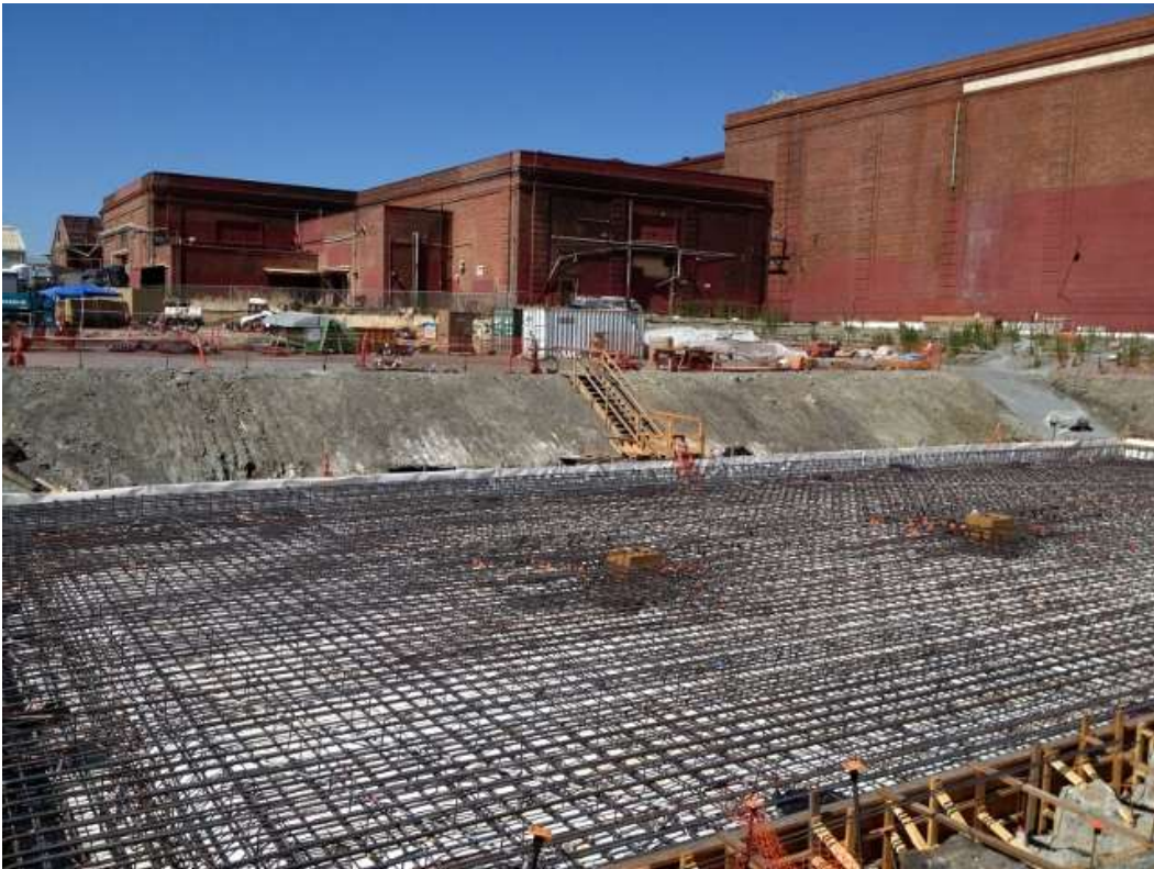
Figure 4 – Potrero Switchyard rebar and grounding work. View northeast, July 29, 2015.
