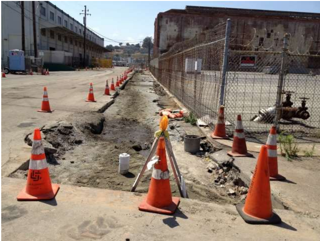
Figure 3 – Duct Bank South work area on 23 rd Street. View west, August 7, 2015.
