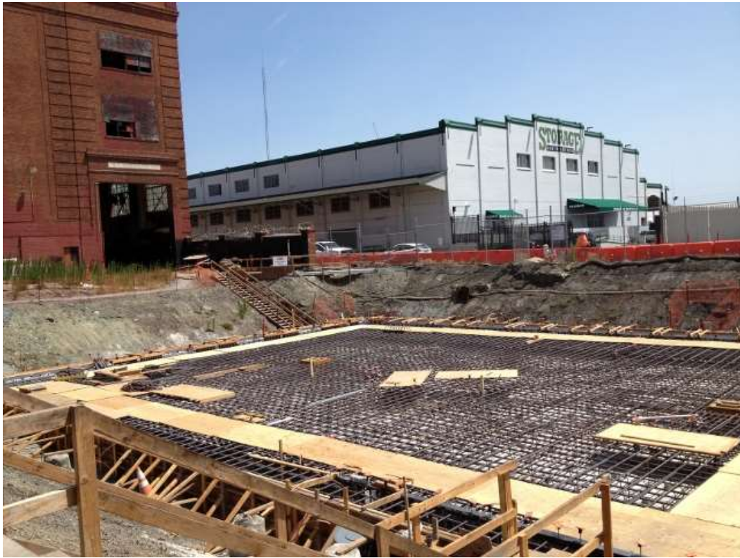
Figure 4 – Potrero Switchyard embeds installation. View southeast, August 7, 2015.
