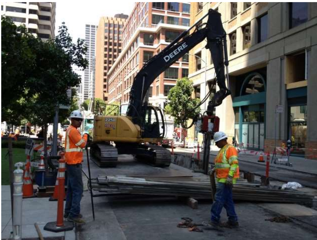
Figure 2 – Removing shoring from trench on Spear Street. View west, August 7, 2015.
