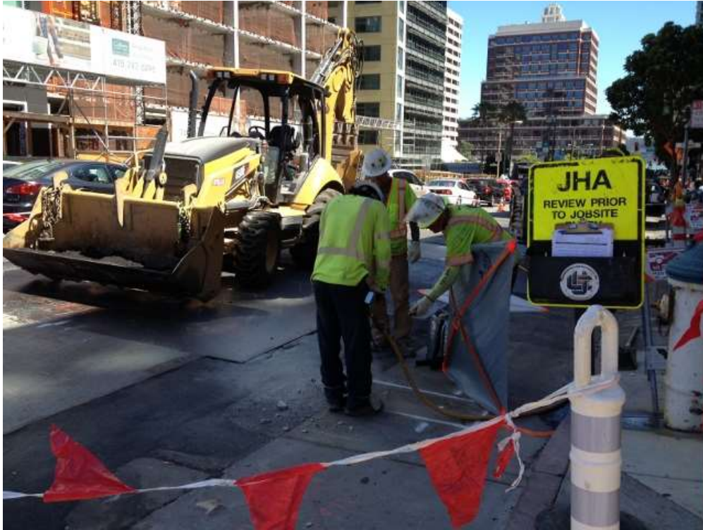
Figure 1 – Jackhammering on Folsom Street near Fremont Street. View northwest, August 14, 2015.
