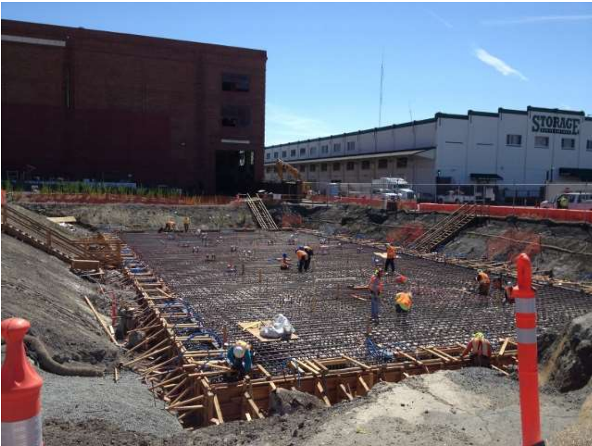
Figure 5 – Potrero Switchyard embeds installation. View southeast, August 14, 2015.
