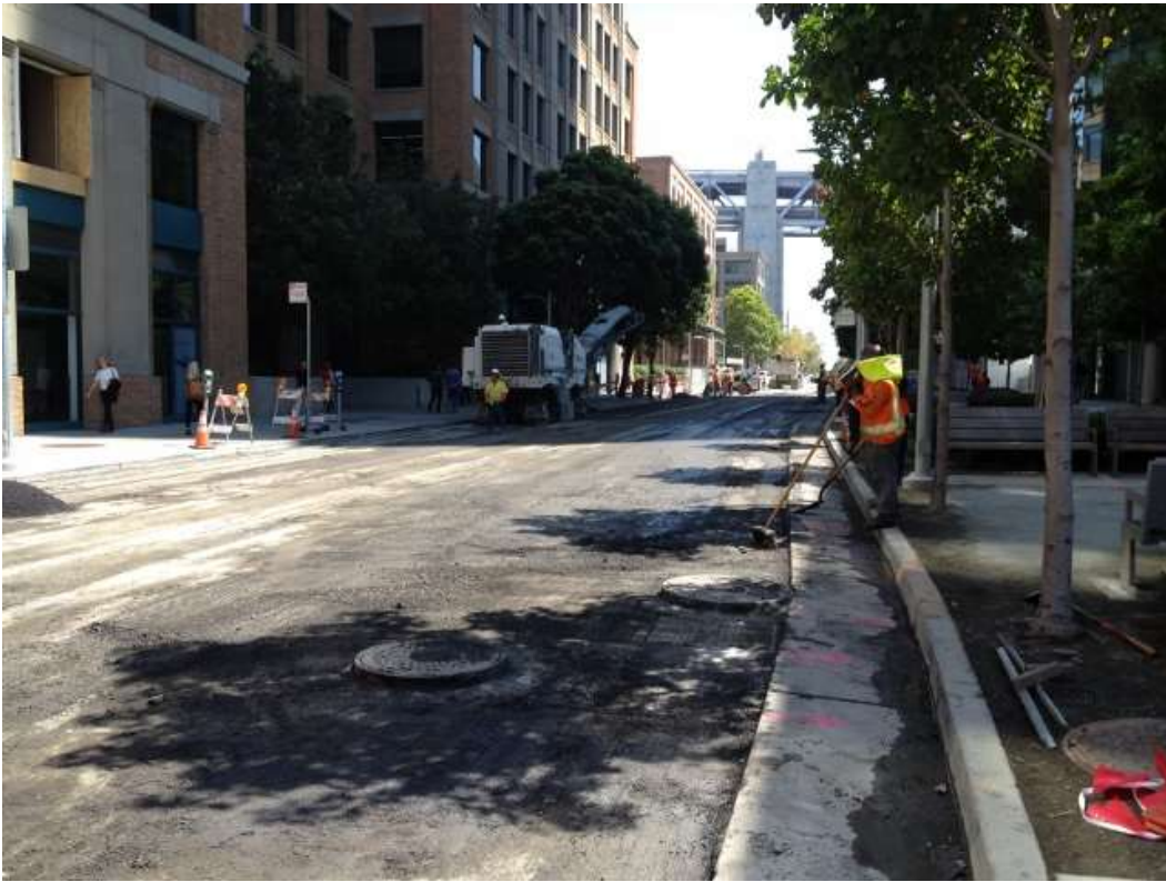
Figure 3 – Grinding asphalt and removing pavement on Spear Street. View east, August 25, 2015.
