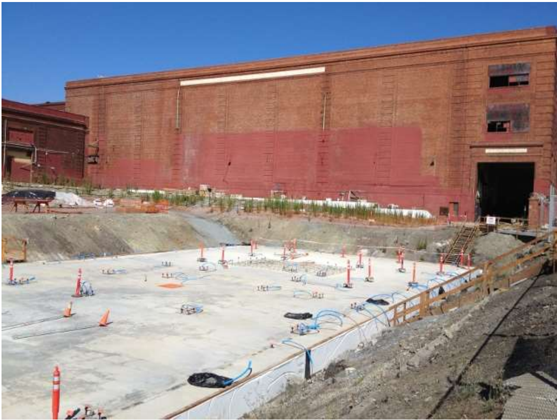
Figure 5 – Potrero Switchyard building foundation concrete pad. View northeast, August 25, 2015.
