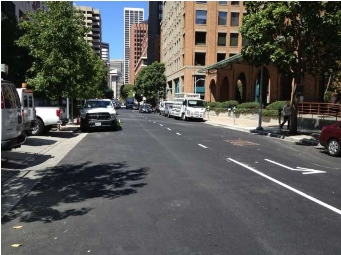
Figure 4 – Spear Street paved and temporarily striped. View west, September 1, 2015.
