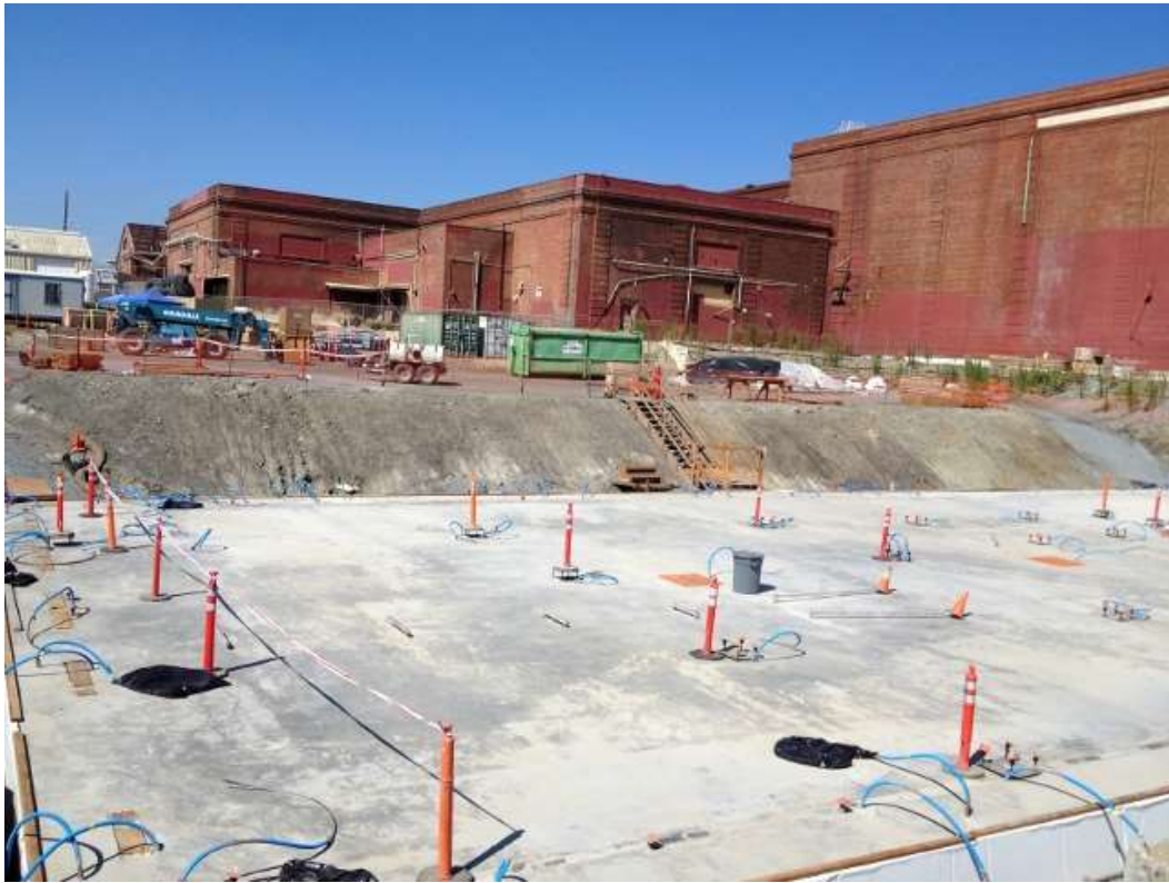
Figure 5 – Potrero Switchyard GIS building foundation concrete pad. View north, September 1, 2015.
