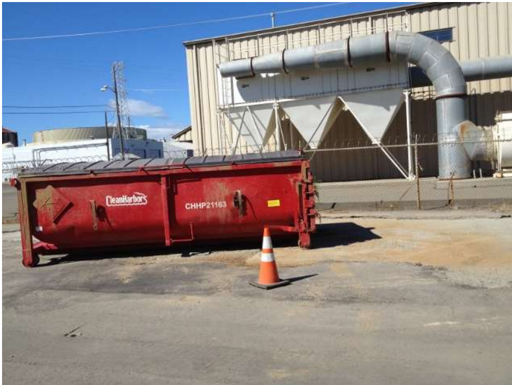
Figure 4 – Dried spoils spill from roll off bin on 23 rd Street. View north, October 1, 2015.
