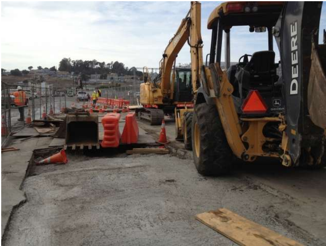
Figure 3 – Trench work on 23 rd Street. View west, October 15, 2015.
