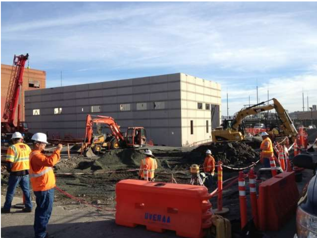
Figure 4 – Potrero Switchyard work. View southeast, November 17, 2015.
