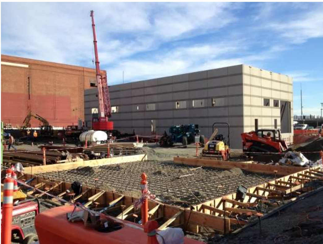
Figure 2 – Work at Potrero Switchyard. View southeast, December 1, 2015.
