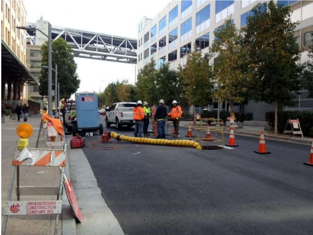
Figure 1 – Crew working in vault on Spear Street. View east, December 1, 2015.
