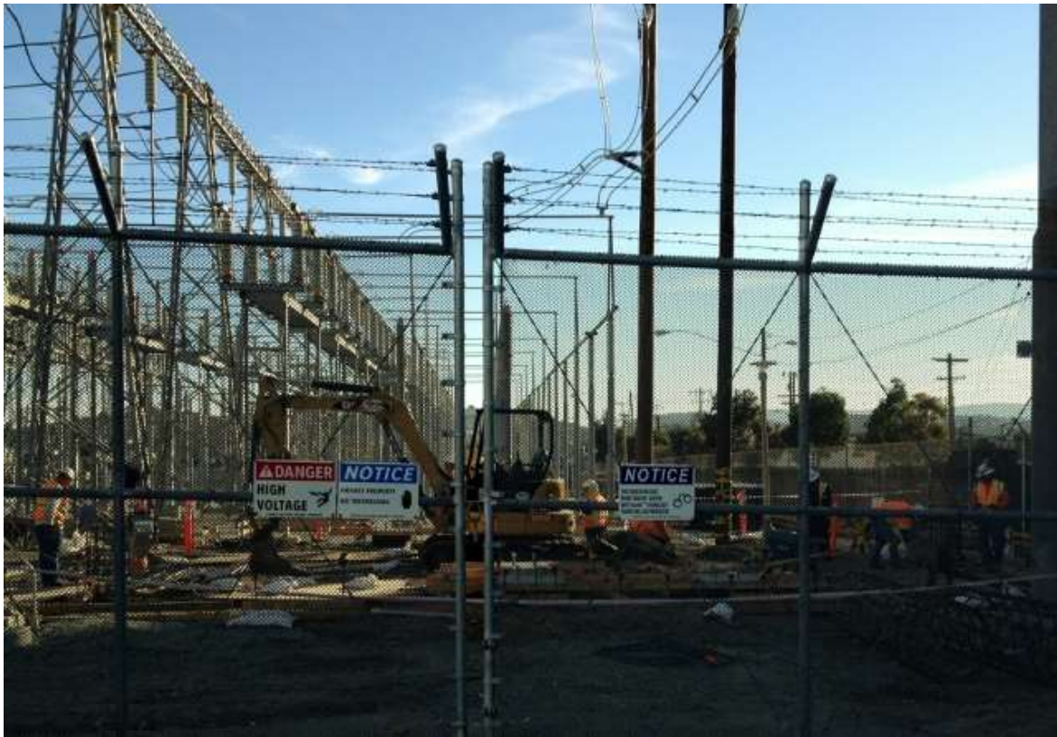
Figure 5 – Crews working in adjacent substation. View south, December 1, 2015.
