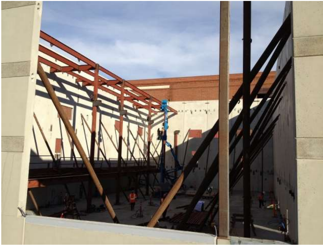
Figure 3 – Crews working in GIS building at Potrero Switchyard. View east, December 1, 2015.
