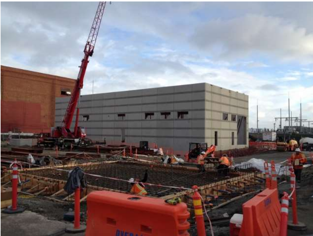
Figure 2 – Work on reactor pad in Potrero Switchyard. View southeast, December 11, 2015.
