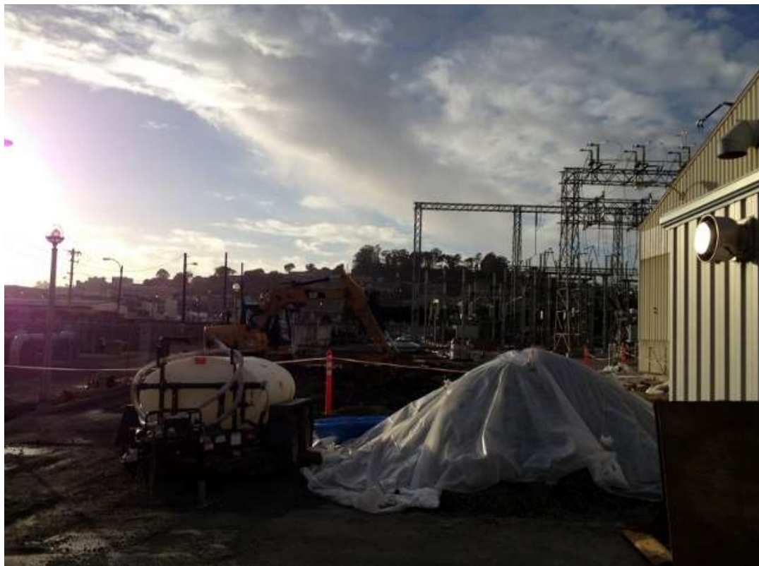
Figure 4 – Excavation work in substation adjacent to Potrero Switchyard. View west, December 11, 2015.
