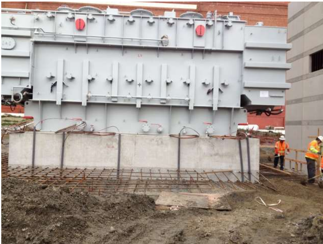
Figure 4 – APEC installing rebar at the transformer pad. View south, January 28, 2016.
