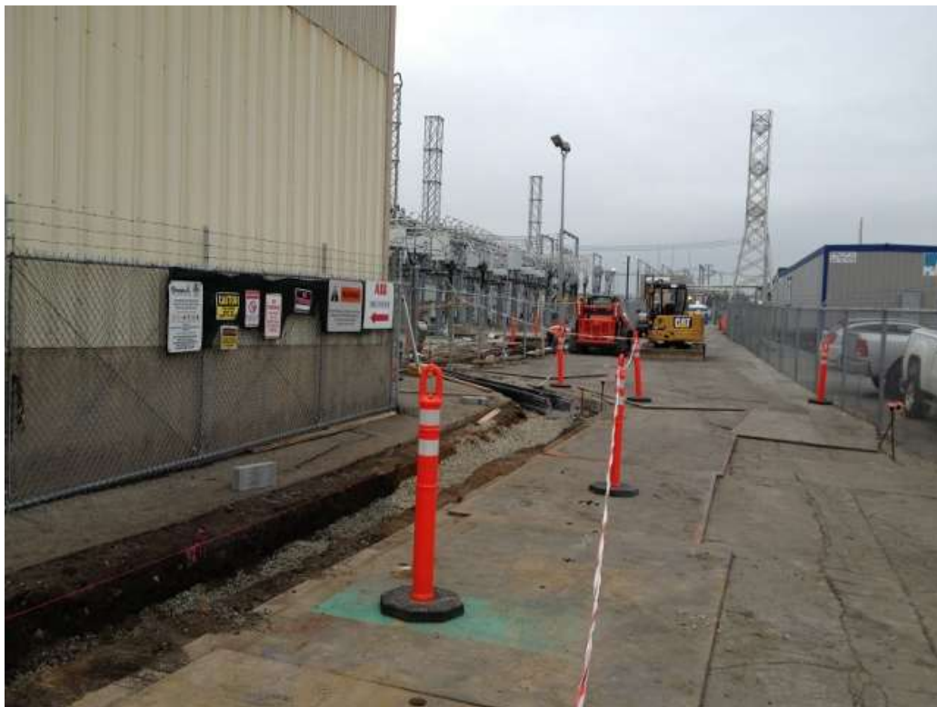
Figure 2 – Crews excavating a trench for GIS building power cable. View north,
