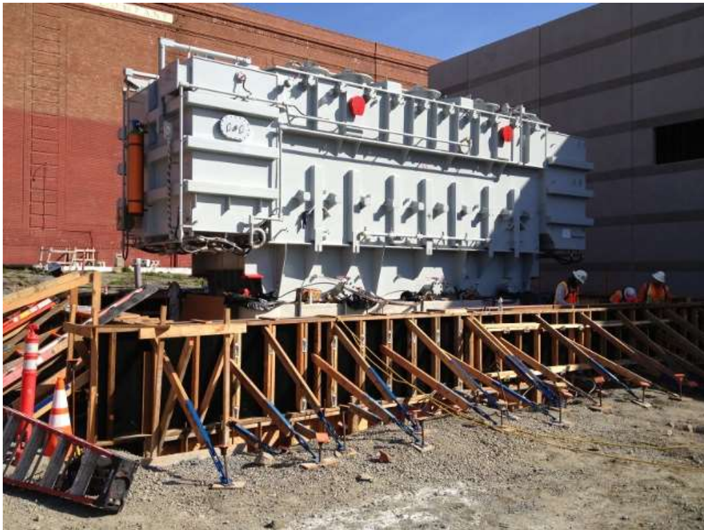
Figure 2 – Crews constructing containment walls around the transformer (SPCC). View southeast, February 24, 2016.
