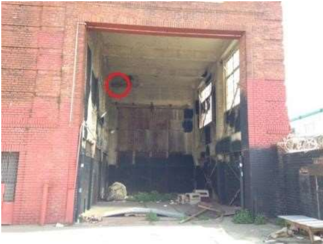
Figure 4 – Common raven nest start in Station A building adjacent to southeast corner of Potrero Switchyard. View east, March 2, 2016. Photo courtesy of PG&E.
