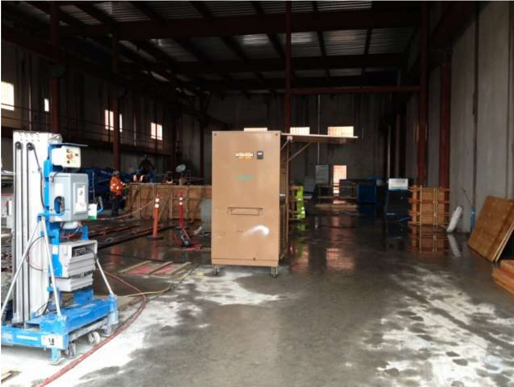
Figure 1 – Crews working in the GIS building. View east, March 9, 2016.
