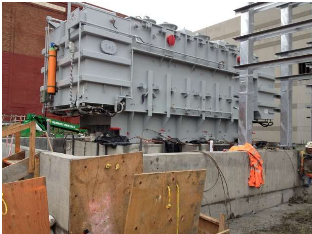
Figure 4 – Crews assembling the transformer. View southeast, March 9, 2016.
