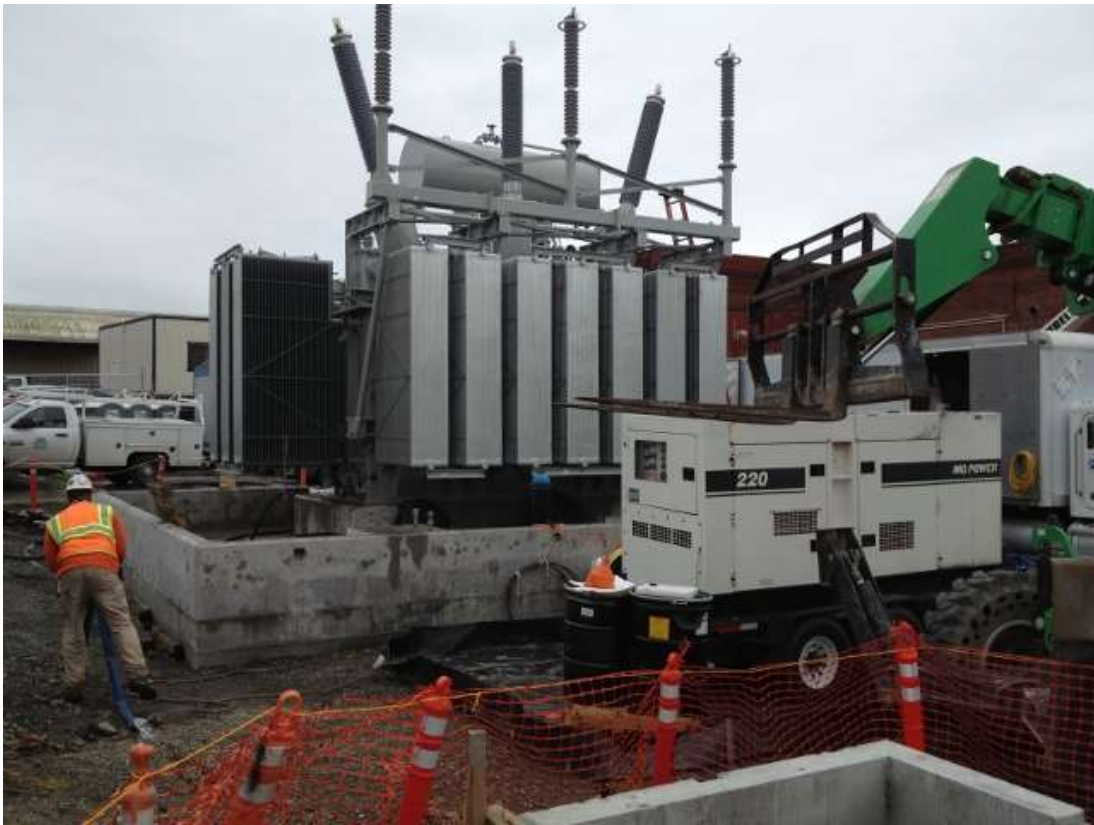
Figure 3 – Crews assembling the reactor. View north, March 9, 2016.
