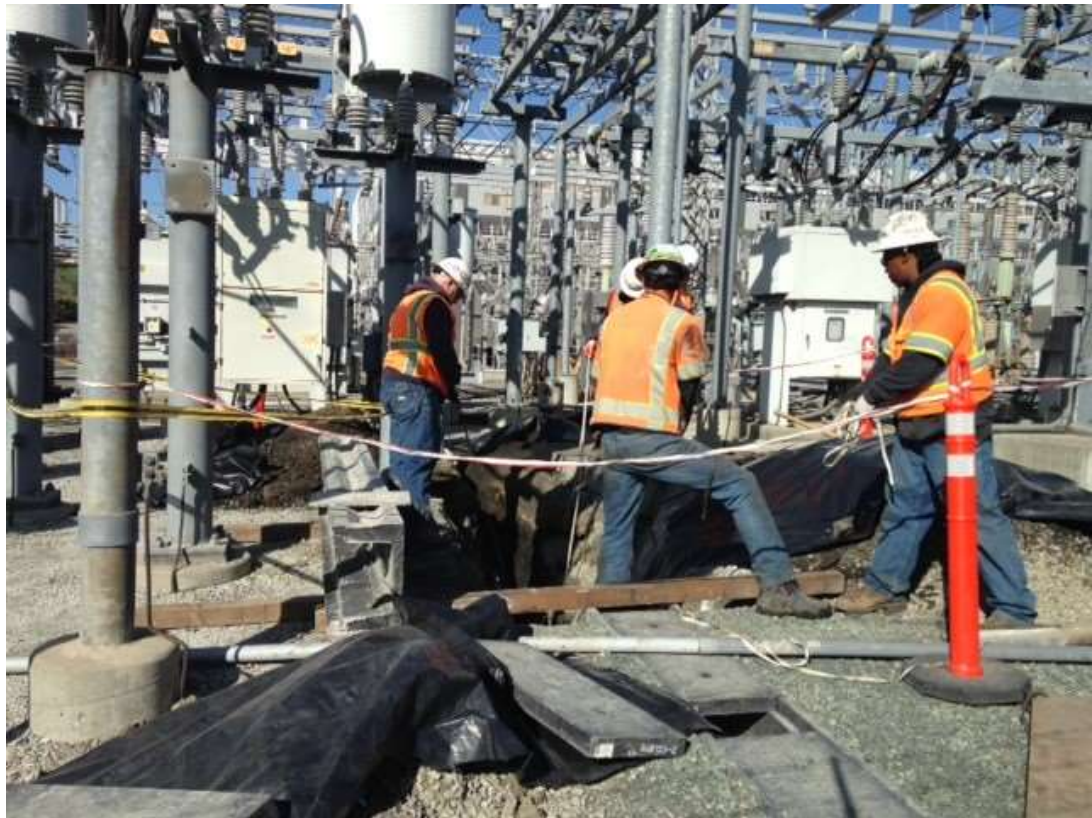
Figure 4 – Crews excavating in substation. View west, March 15, 2016. Photo courtesy of PG&E.
