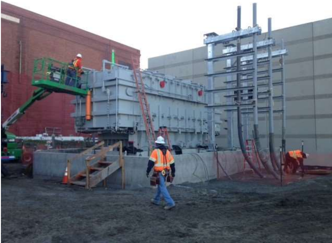
Figure 3 – Crews assembling the transformer. View southeast, March 16, 2016. Photo courtesy of PG&E.
