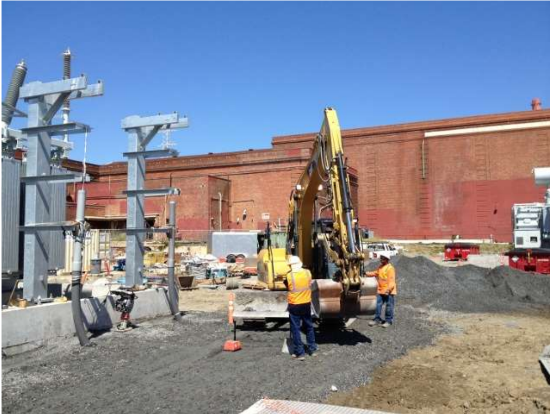
Figure 1 – APEC compacting backfill around the reactor pad. View east, May 9, 2016.
