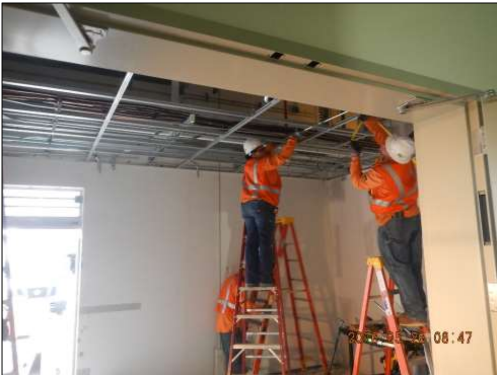
Figure 2: MEI worked on wiring at Potrero Switchyard, May 26, 2016. Photo courtesy of PG&E.
