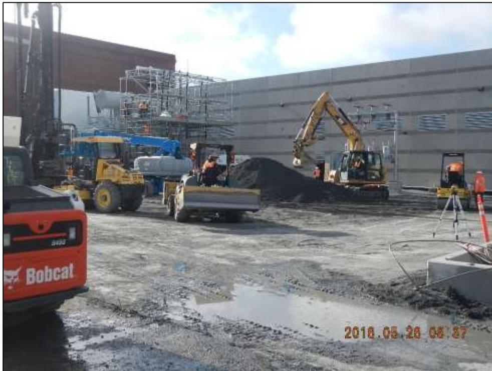
Figure 1: APEC backfilled at Potrero Switchyard, May 26, 2016. Photo courtesy of PG&E.
