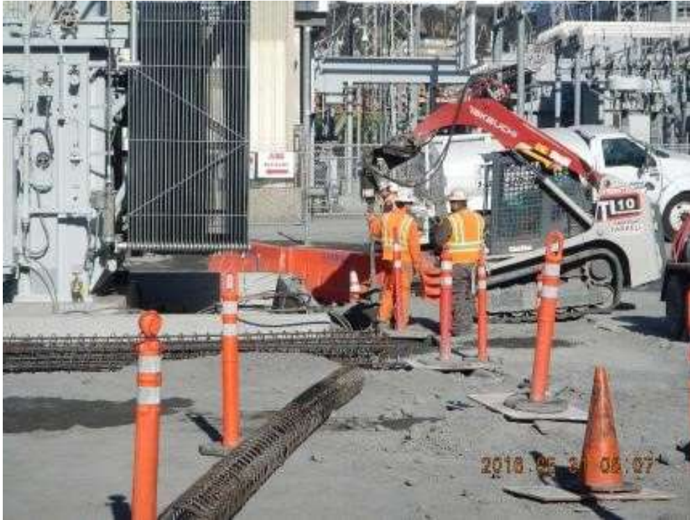
Figure 1: Farrell drilled at the Potrero Switchyard, May 31, 2016. Photo courtesy of PG&E.
