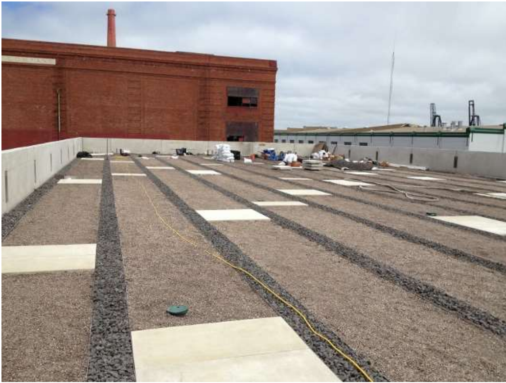
Figure 3: Landscaping work on the GIS building roof, June 9, 2016.
