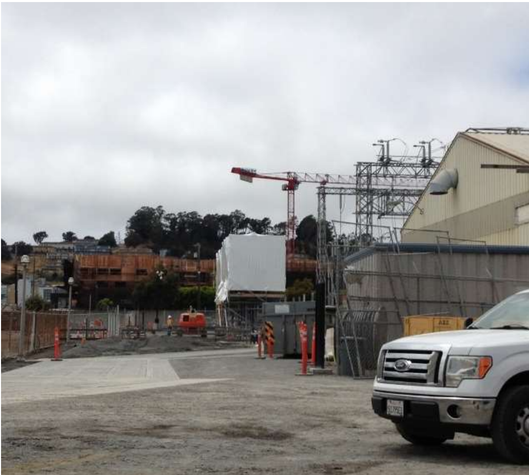
Figure 4: Substation work around the 115 kV bus, June 9, 2016.
