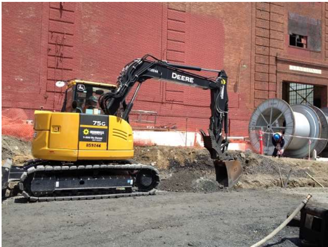
Figure 2: Proven excavated for the perimeter wall, June 9, 2016.
