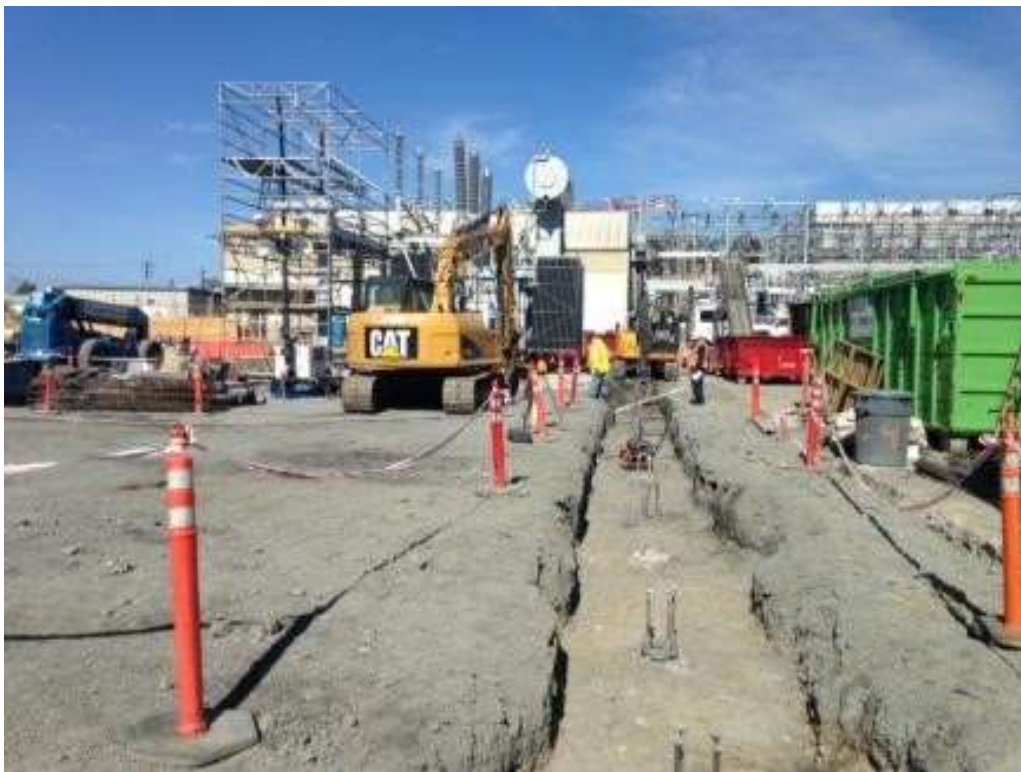
Figure 2: Proven excavated for the perimeter wall, June 14, 2016. Photo courtesy of PG&E.
