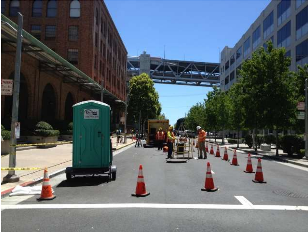
Figure 1: Preparing for cable pull into the vault on Spear Street, July 12, 2016.
