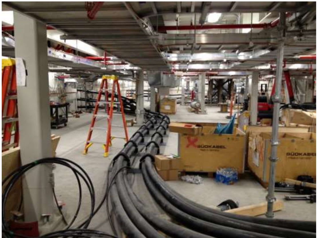
Figure 4: Cable pulled through basement of GIS building in Potrero Switchyard, July 26, 2016.
