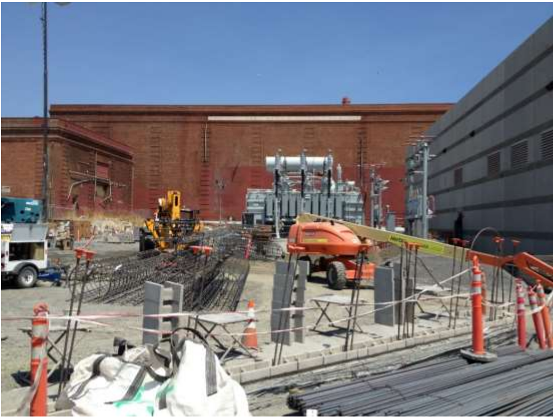
Figure 3: Perimeter wall being installation at Potrero Switchyard, July 26, 2016.
