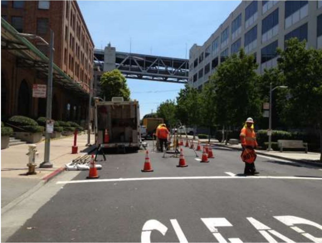
Figure 1: Splicing cable in transition vault on Spear Street, July 26, 2016.
