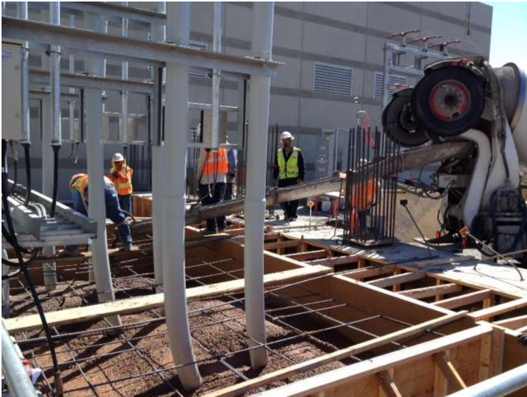
Figure 3: Flowable thermal backfill (FTB) was poured around the transformer, August 9, 2016.
