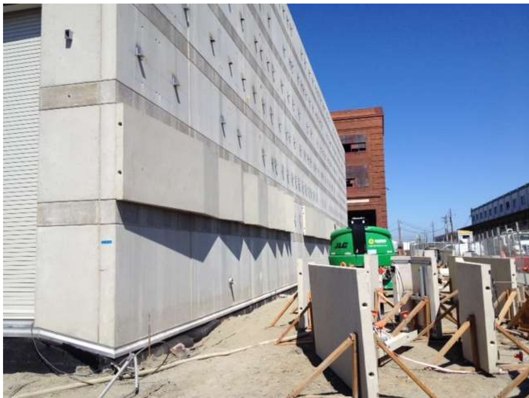
Figure 2: Overaa installed the architectural panels on the GIS building, August 9, 2016.
