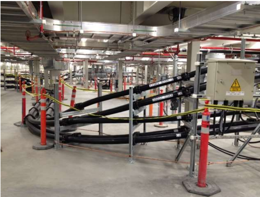
Figure 2 - CCE conducted electrical work in the GIS building, September 1, 2016.
