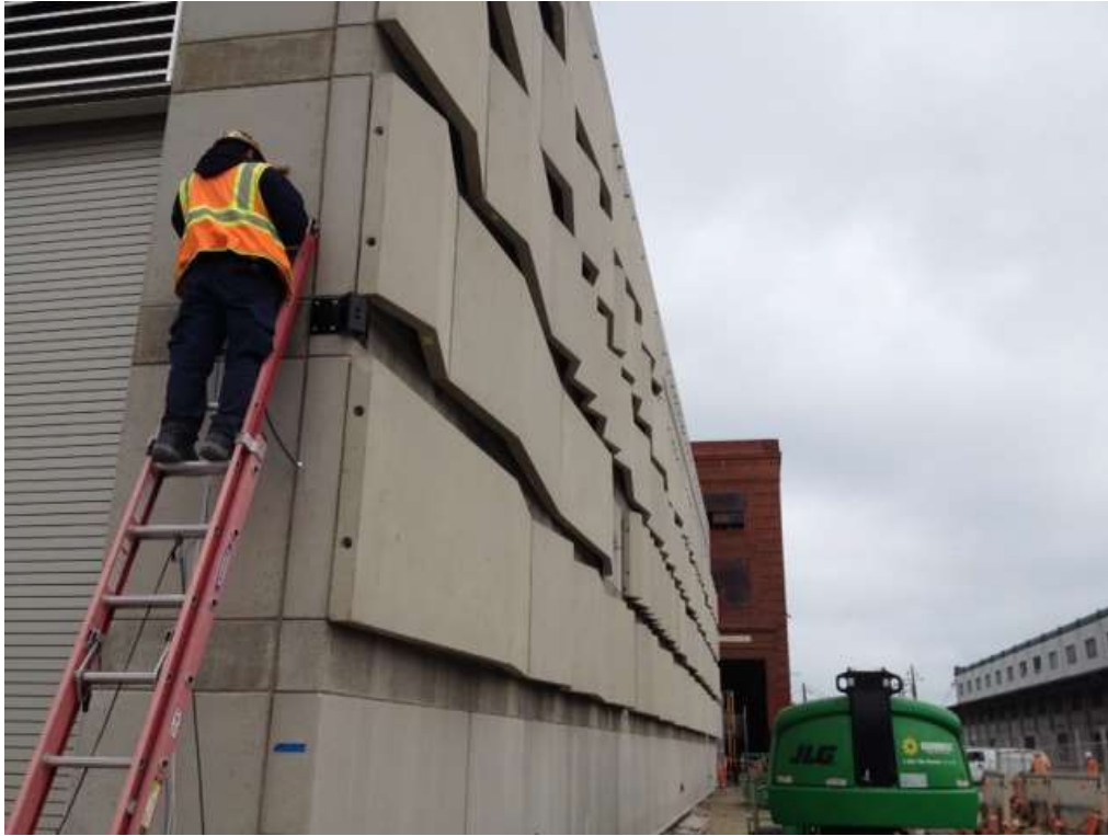
Figure 1 - Overaa installing architectural tiles on GIS building at Potrero Switchyard, September 1, 2016.
