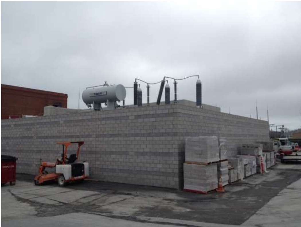
Figure 3 - Spencer Masonry building perimeter wall in Potrero Switchyard, September 1, 2016.
