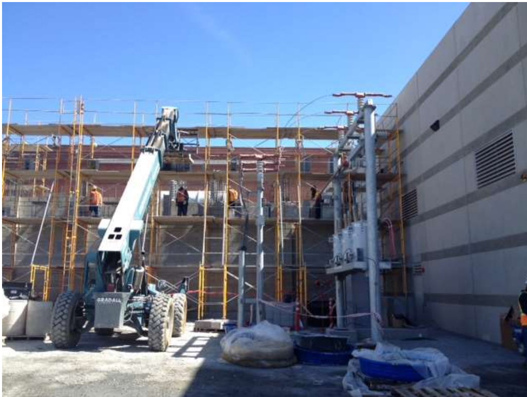
Figure 2 – Spencer Masonry building fire wall on west side of transformer, September 21, 2016.
