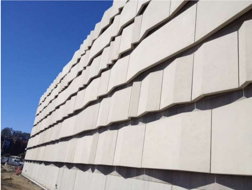
Figure 1 - Architectural tiles on GIS building at Potrero Switchyard being repaired, September 21, 2016.
