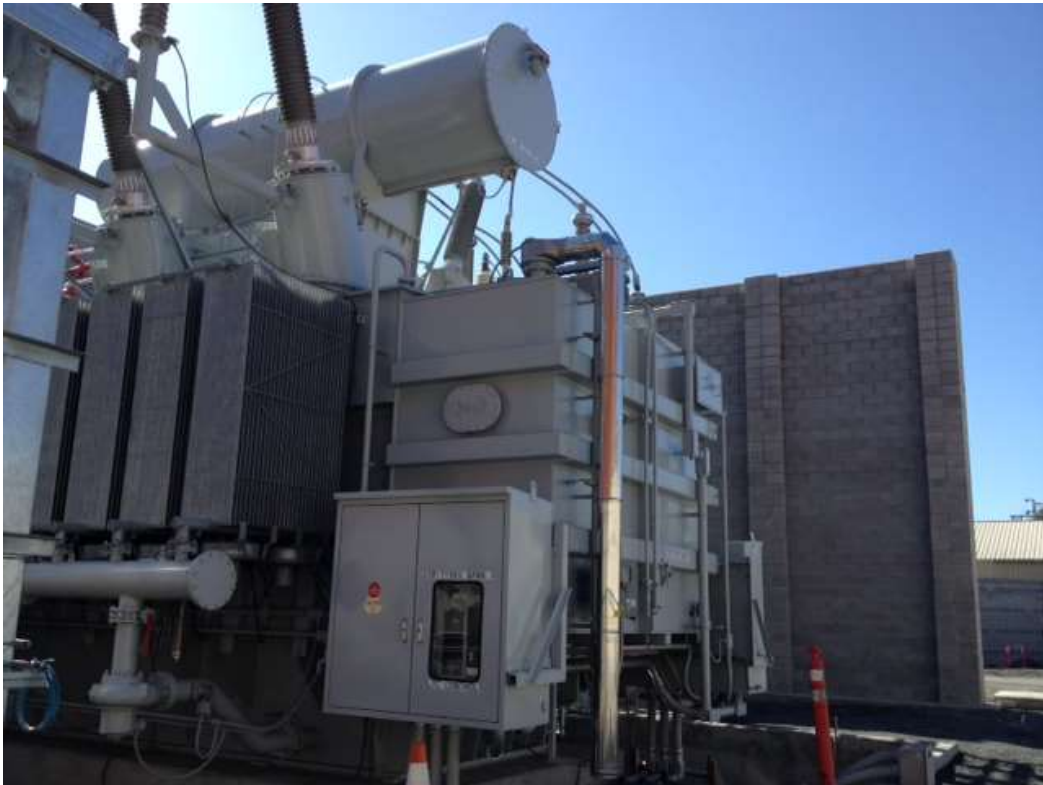
Figure 3 – Wall around the transformer completed and all electrical work done, October 26, 2016.
