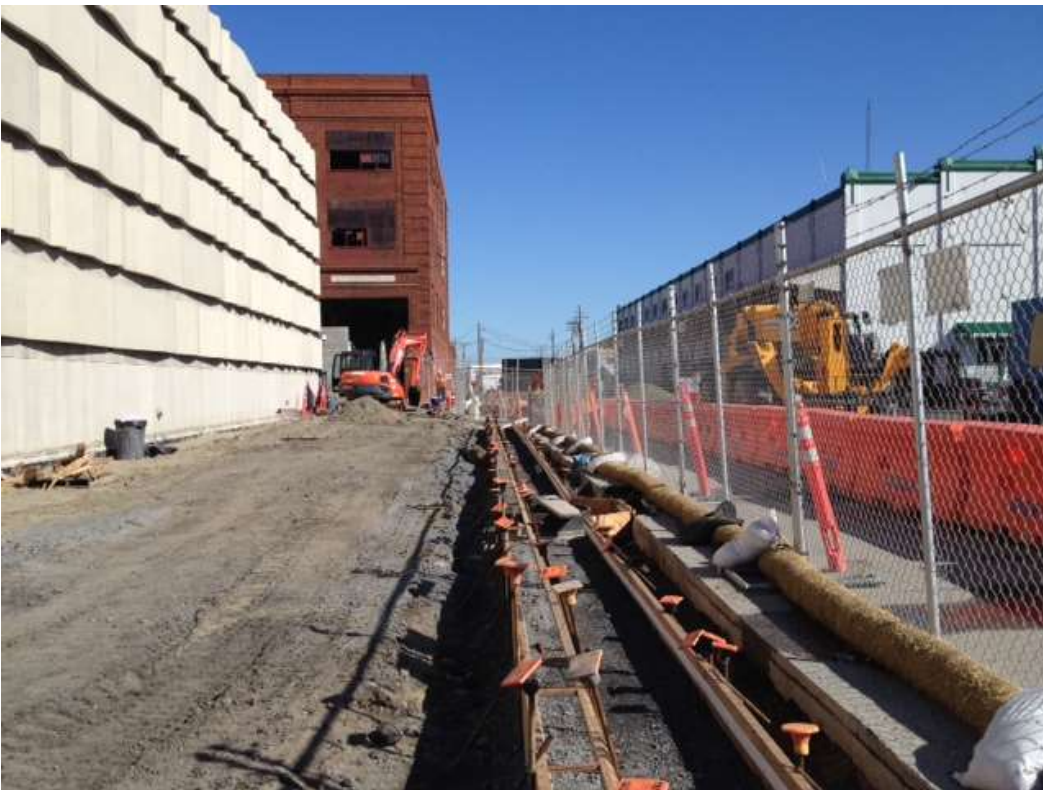
Figure 4 – Sidewalk, curb, and drainage work along 23 rd Street, October 26, 2016.
