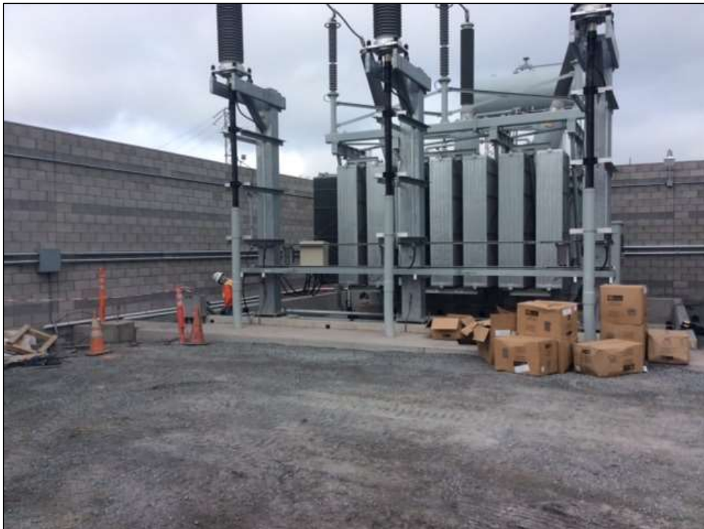
Figure 2 – APEC installing grating in reactor containment, November 15, 2016. Photo courtesy of PG&E.
