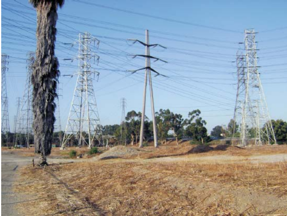
View of Site Looking South
