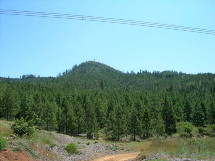
Existing Facilities—Distance View
