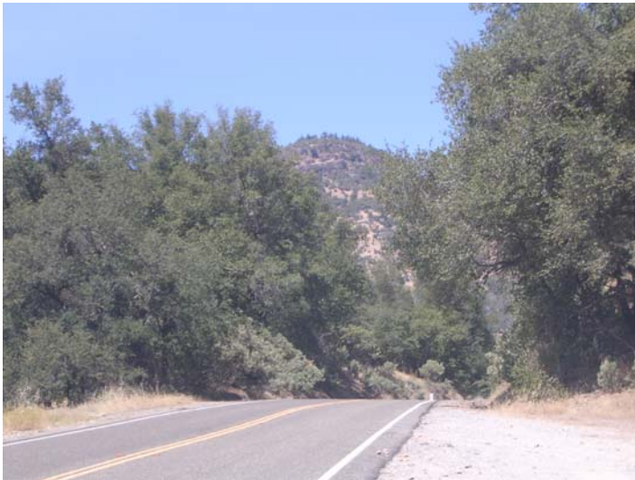
Existing Facilities—Distance View
