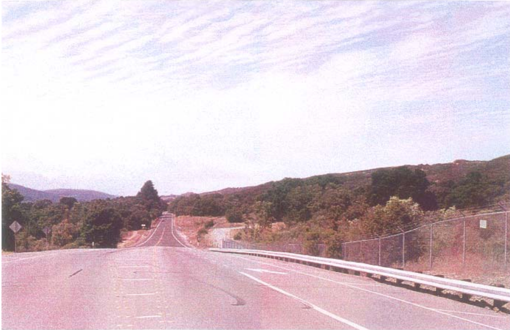
Existing view from northbound Cañada Road near Edgewood Road
