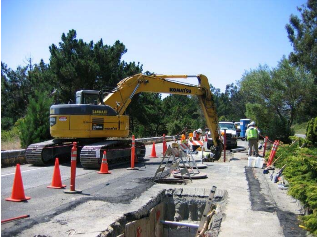
Figure 3 – Excavation of Manhole #41 stubouts along San Bruno Ave, Segment 3, August 12, 2005.
