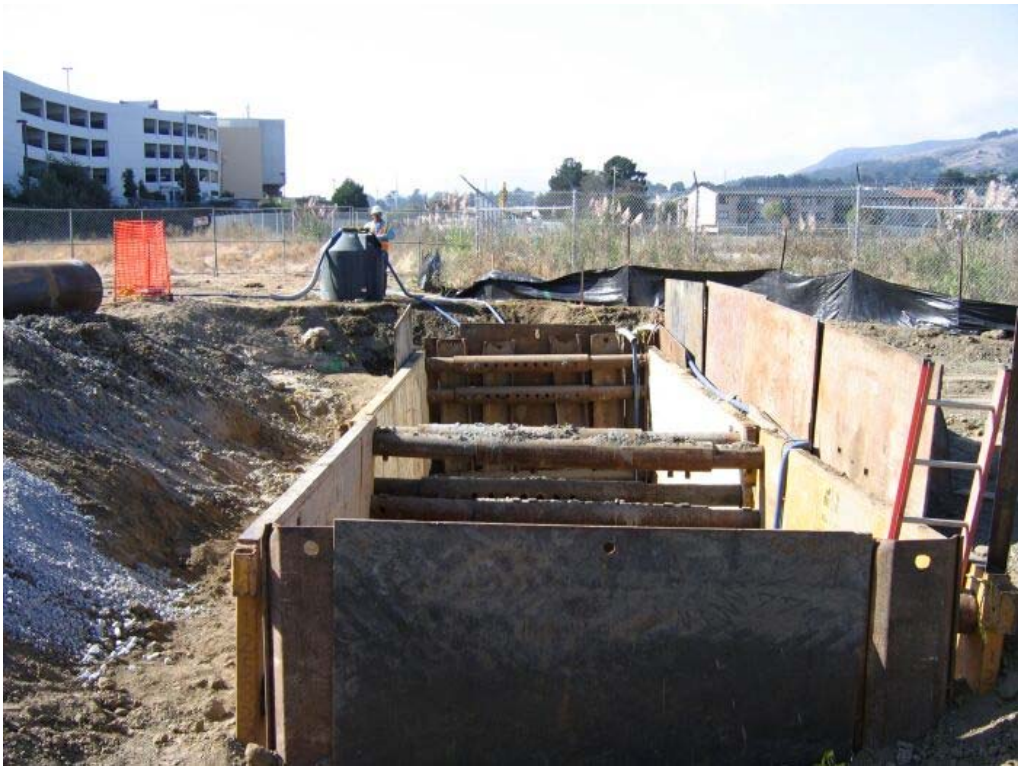
Figure 4 – Bore pit shored on South side of Colma Creek, Segment 4, August 24, 2005
