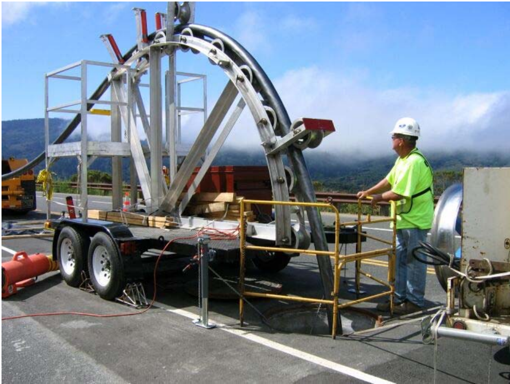
Figure 1 – Crews conducting cable pulling at Manhole #14 on Cañada Road, Segment 1, August 18, 2005
