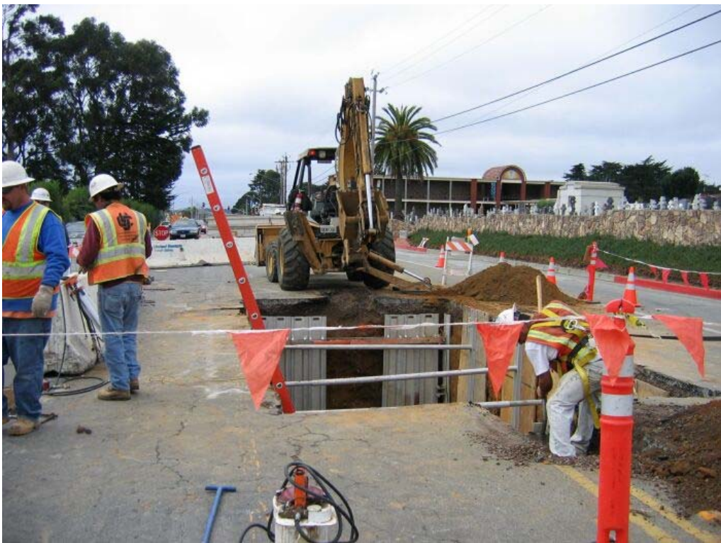
Figure 4 – Excavation and shoring of Manhole #60 on Hillside Drive, Segment 4, September 12, 2005.
