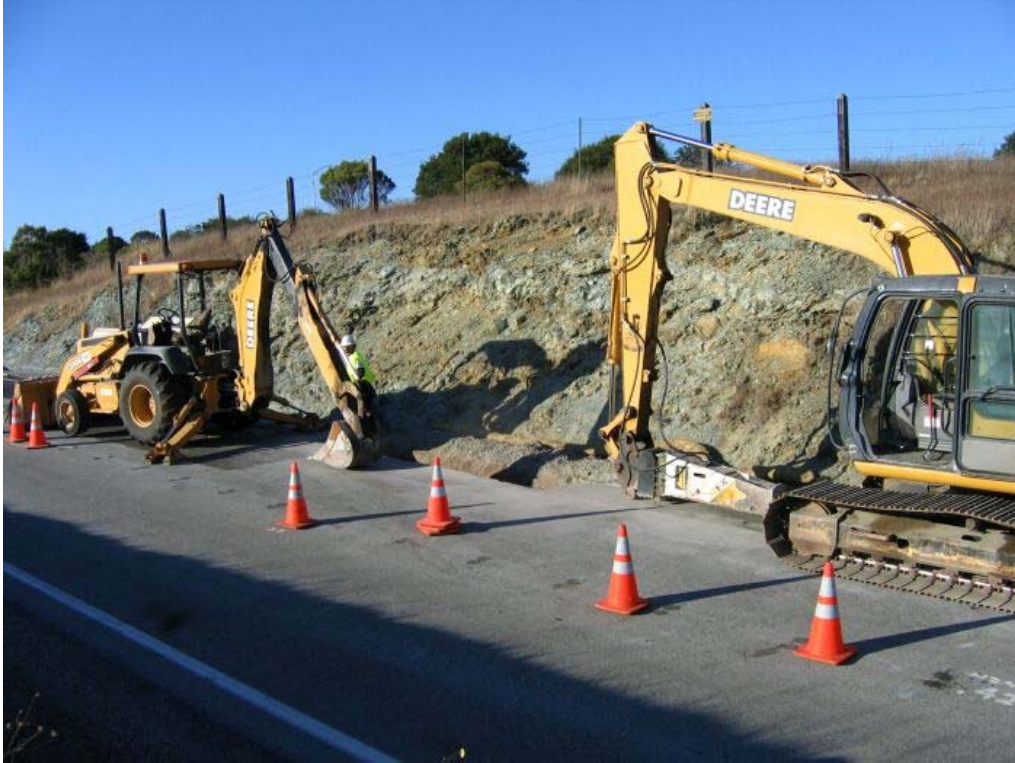
Figure 1 – Crews fixing conduit on south side of Manhole #26, Segment 1, September 12, 2005
