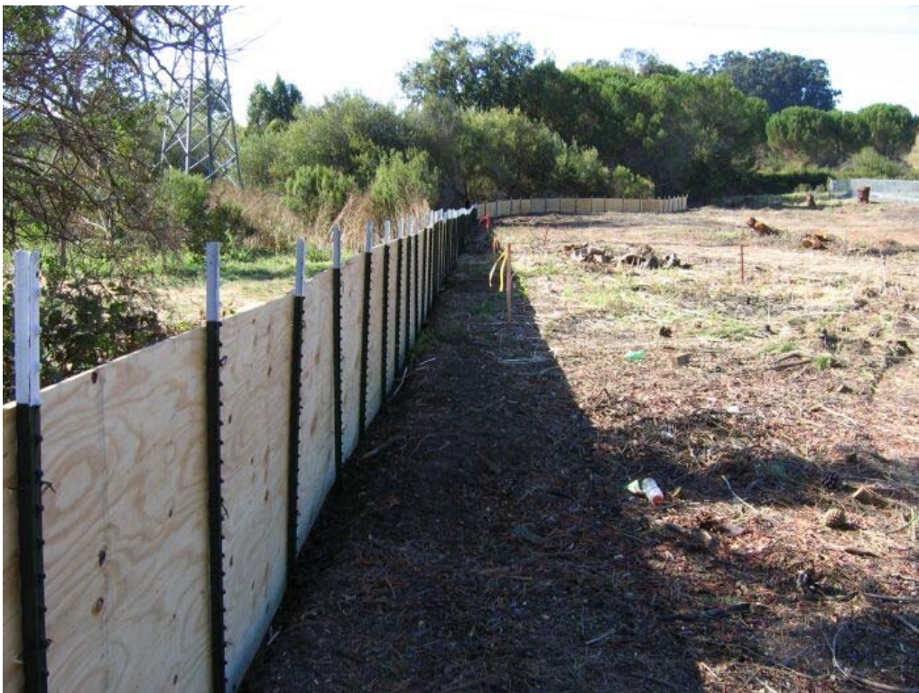
Figure 6 – Plywood fence installation around expansion area at the Jefferson Substation, September 15, 2005.
