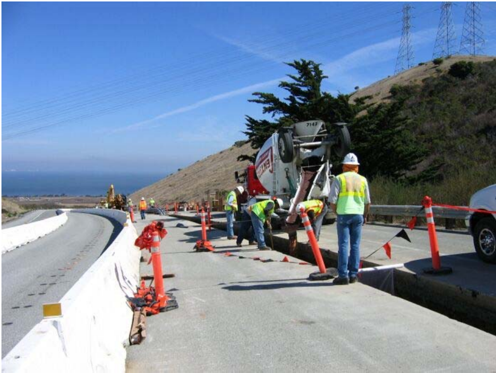
Figure 5 – Trenching activities east of Manhole #74 on Guadalupe Canyon Parkway, Segment 5, September 22, 2005.
