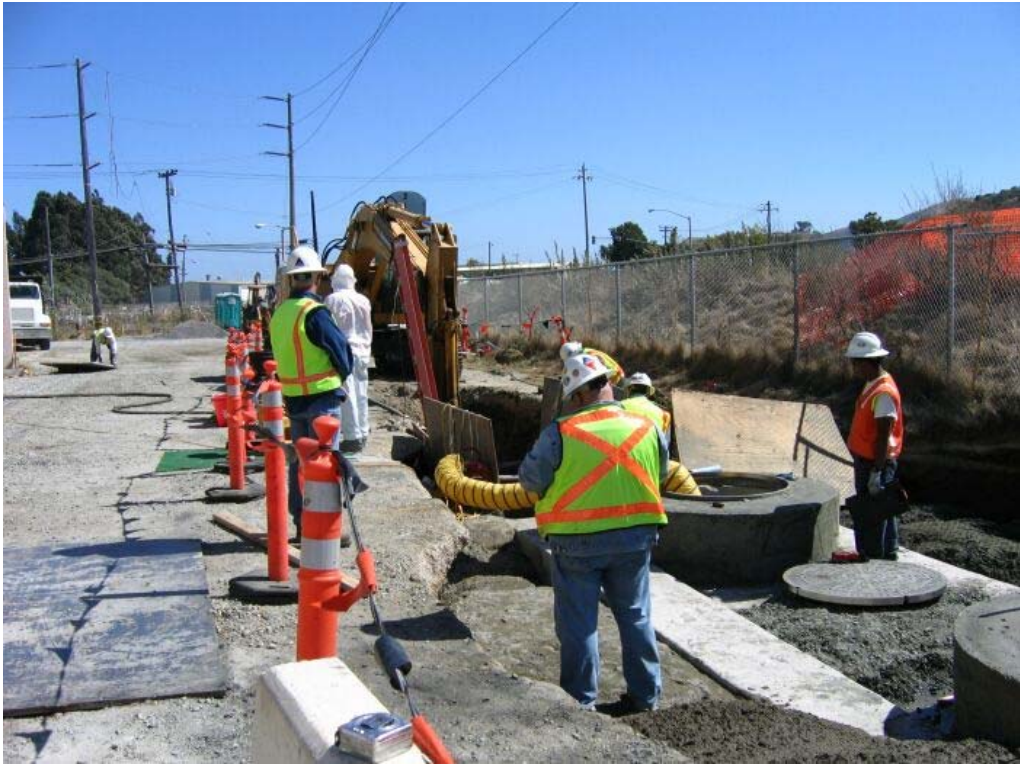
Figure 7 – Crews working at Manhole #79 in the Martin Substation, September 16, 2005.
