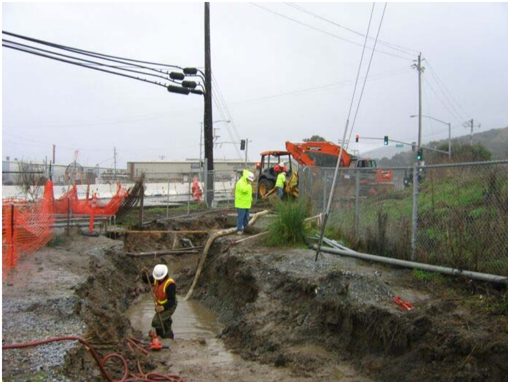
Figure 6 – Excavating trench, removing floated conduit and cement slurry, Martin Substation, December 21, 2005.
