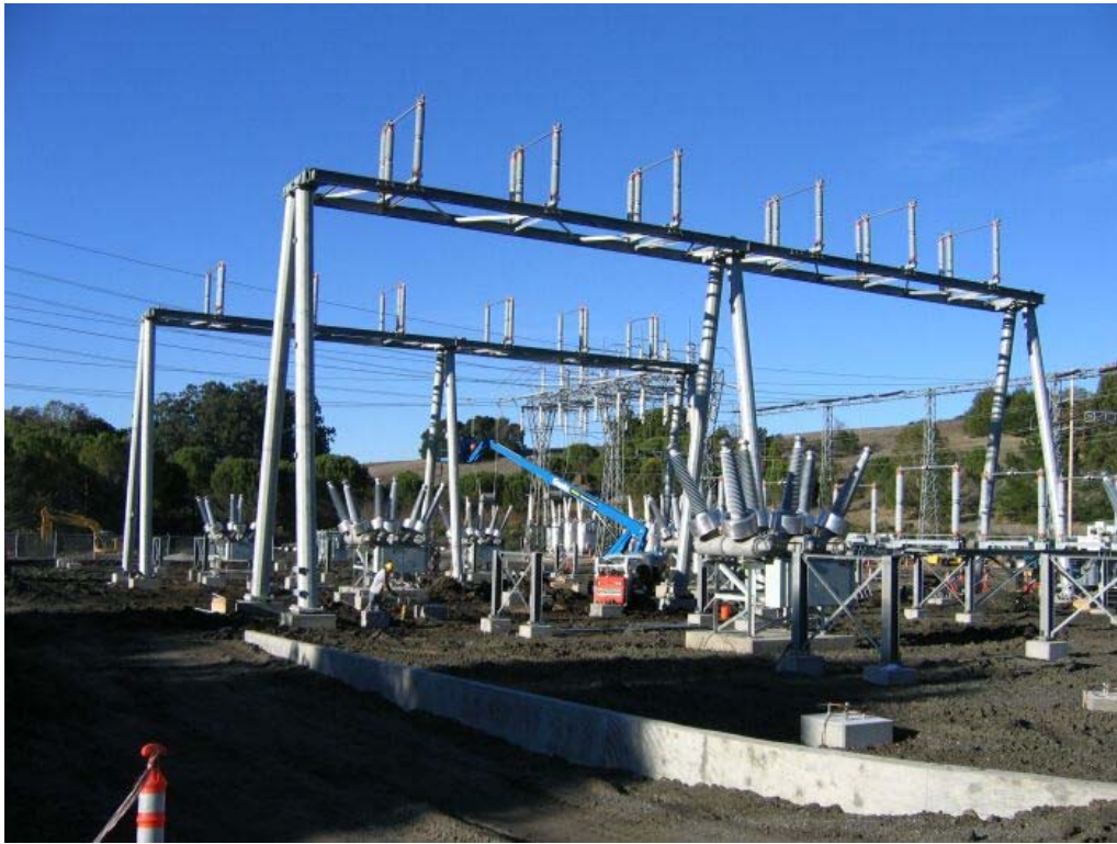
Figure 5 – New structures being worked on in the Jefferson Substation, December 6, 2005.
