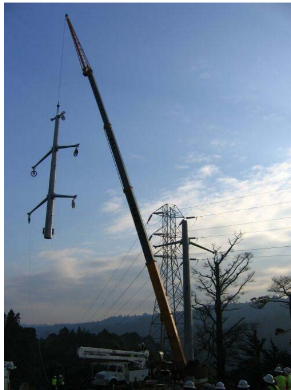
Figure 2 – Crane setting the top of the new Tower #73, Segment 2 Overhead, December 8, 2005.
