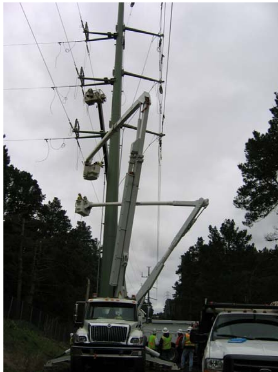
Figure 2 – Crews working at Tower #78, Segment 2 Overhead in the SFPUC watershed, March 16, 2006.
