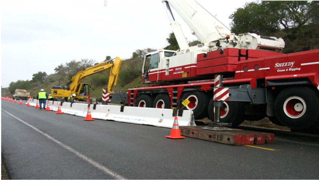
Figure 3 – Crane ready to lower Manhole #9 vault on Segment 1, January 25, 2005.
