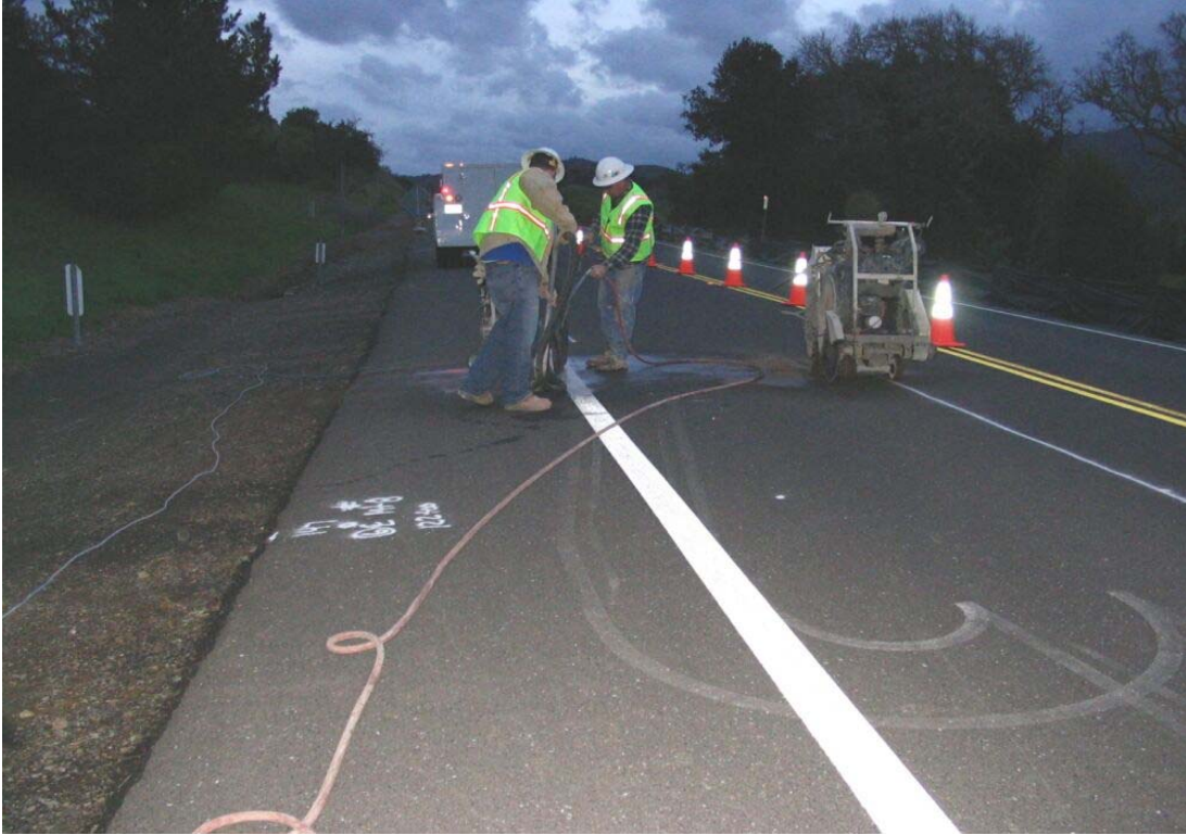
Figure 5 – Crews cutting asphalt for Manhole #8 vault pit on Segment 1, January 27, 2005.
