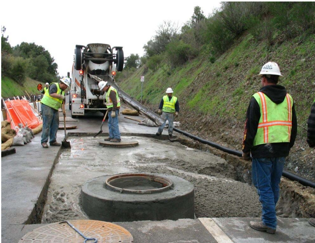
Figure 4 – Crews contouring cement slurry over Manhole #9 vault on Segment 1, January 26, 2005.
