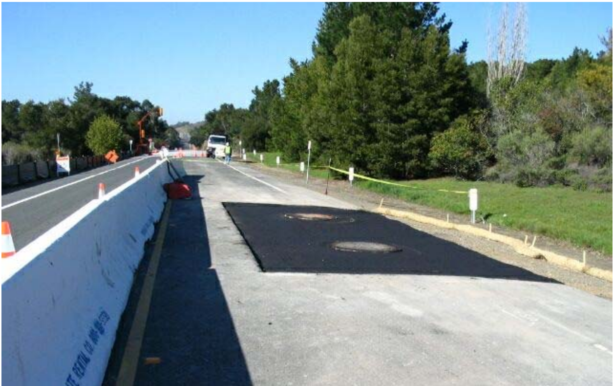
Figure 4 – Manhole #8 paving complete on Segment 1, February 3, 2005.
