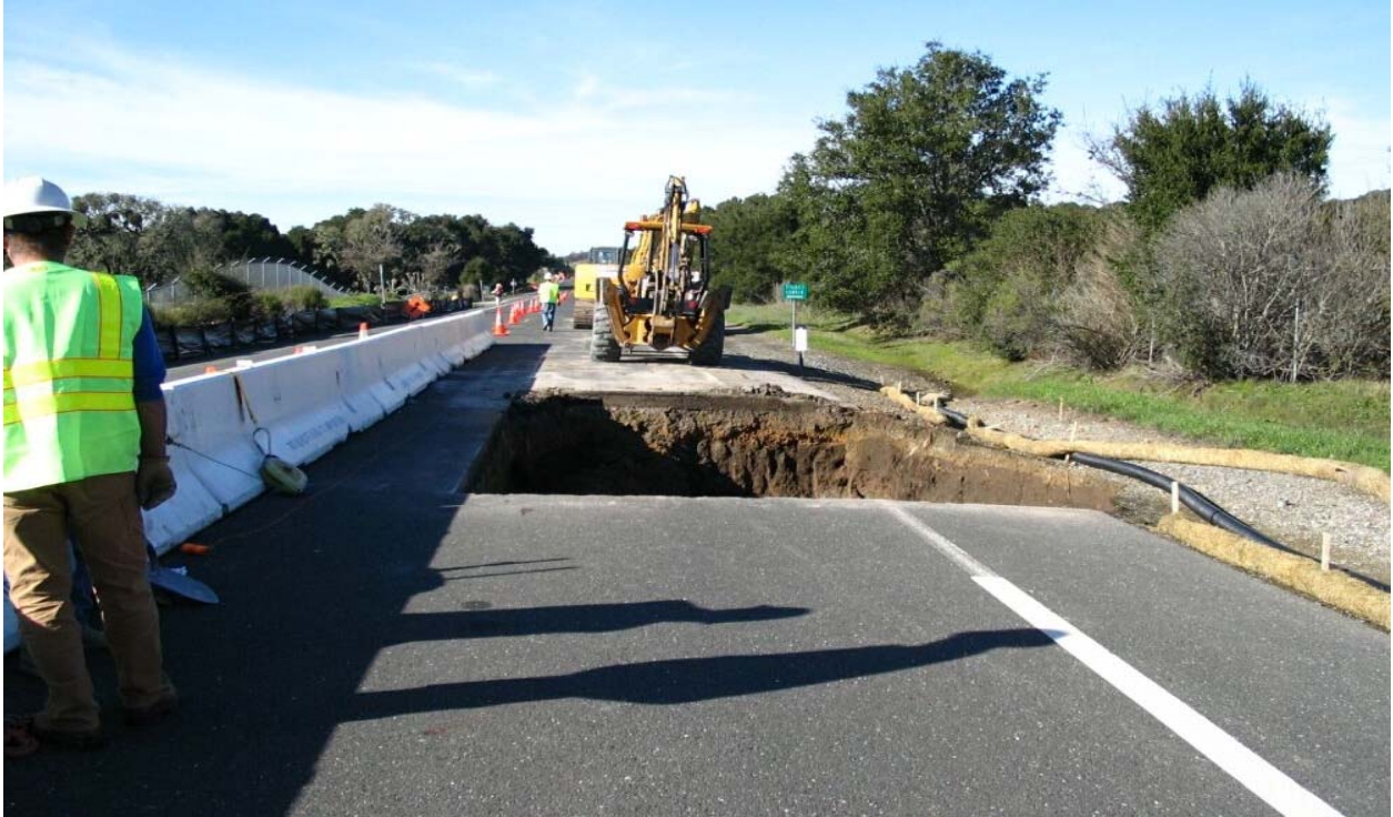
Figure 1 – Crews excavating Manhole #7 vault pit along Cañada Road on Segment 1, January 31, 2005.
