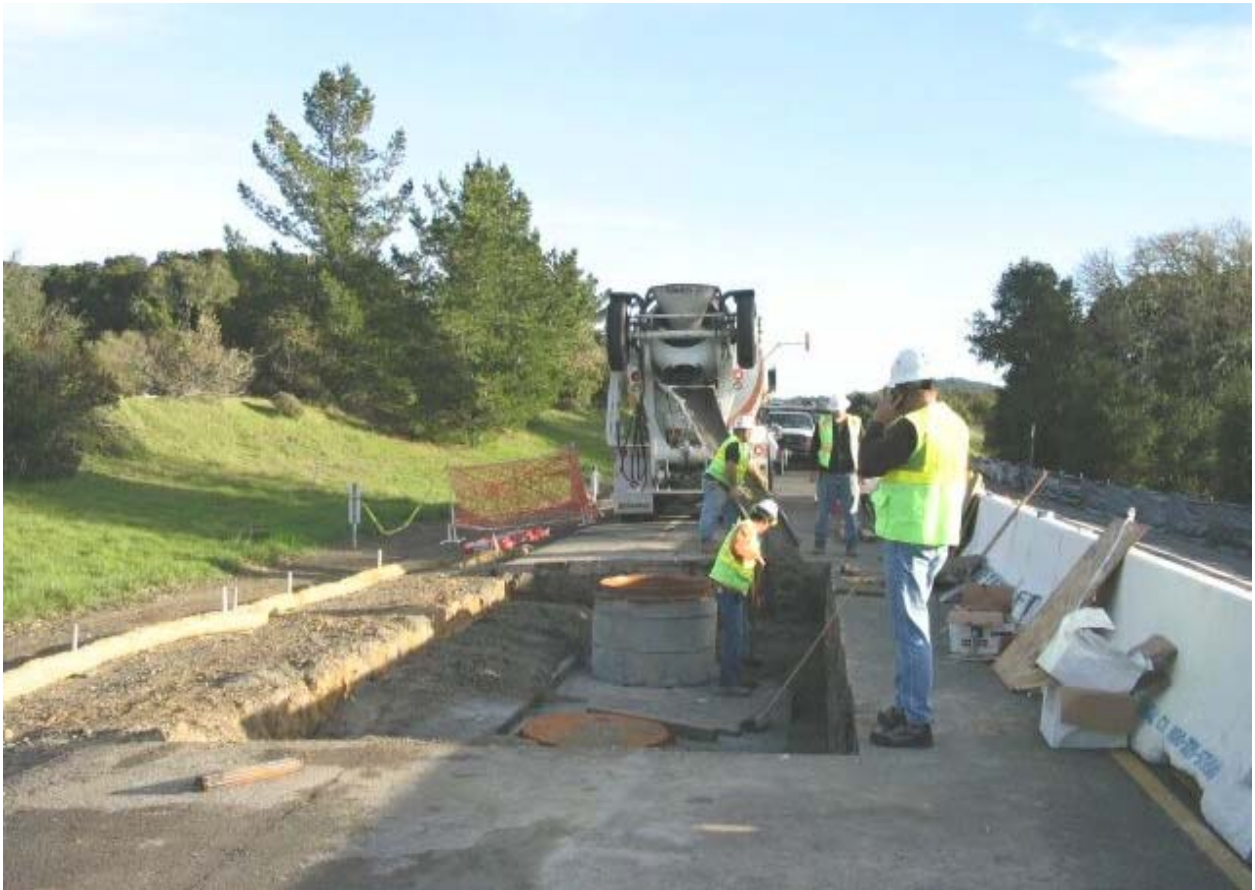
Figure 3 – Crews setting Manhole #8 rings on Segment 1, February 1, 2005.
