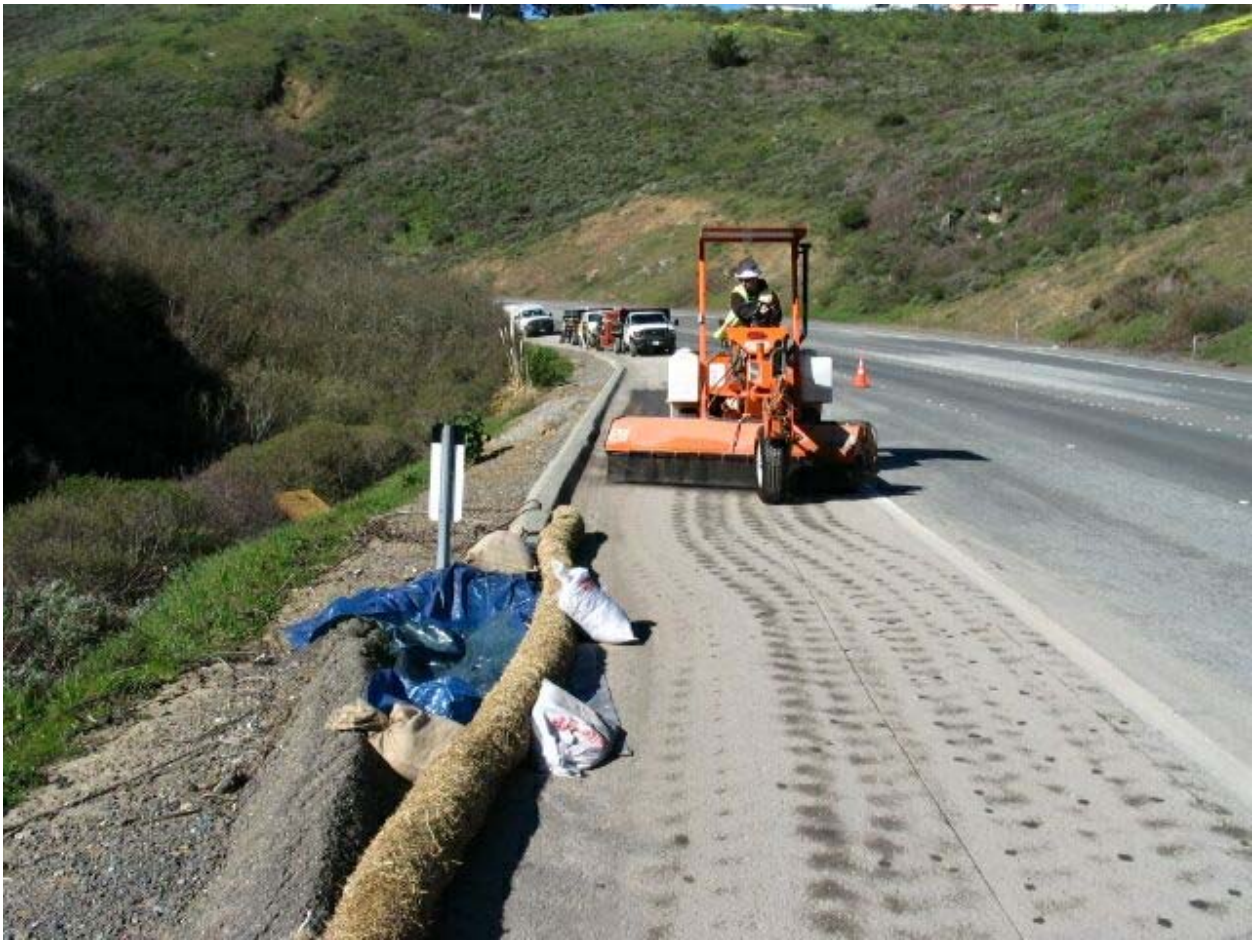
Figure 5 – Crews sweeping road and erosion controls in place on Segment 5, February 2, 2005.
