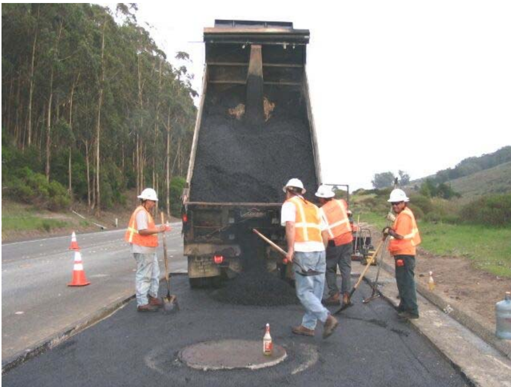
Figure 6 – Manhole #68 paving complete on Segment 5, February 11, 2005.
