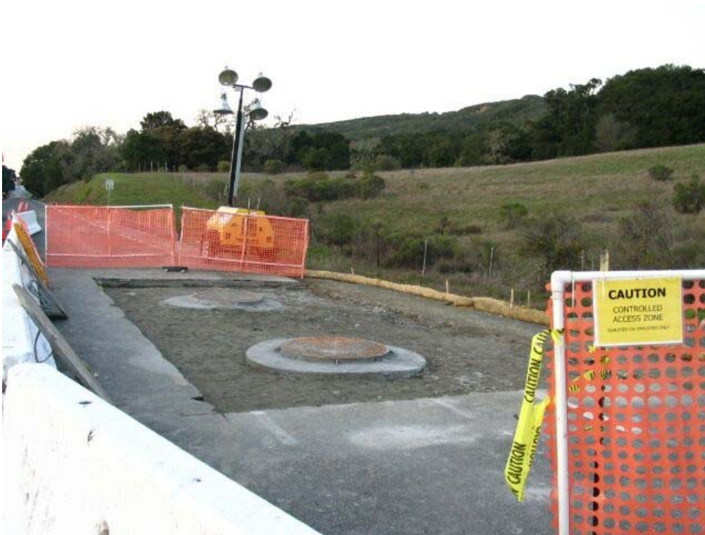
Figure 2 – Manhole #4 on Segment 1, February 9, 2005.
