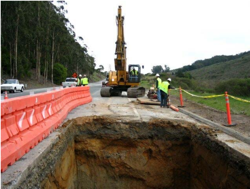
Figure 5 – Preparing for shoring to arrive at MH #68 on Segment 5, February 8, 2005.
